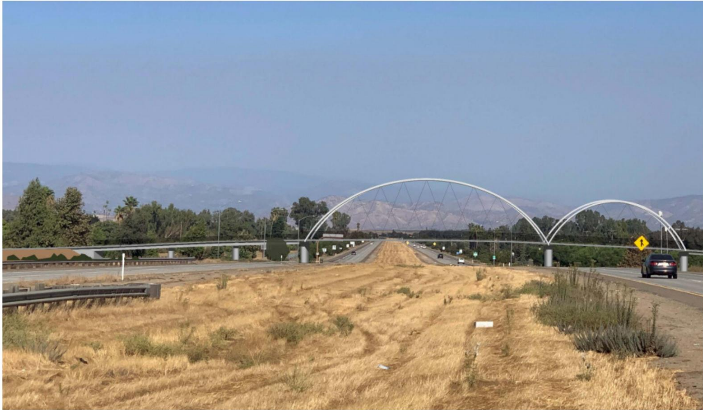
State Route (SR) 168 Enterprise Canal Pedestrian Bridge Project City of Clovis, CA Figure 2.2.1-1
