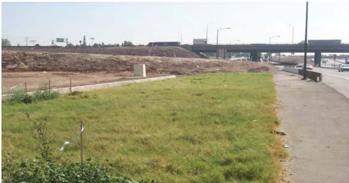
Figure 1-2. Biofiltration Strip (District 7, I-605/SR-91)
