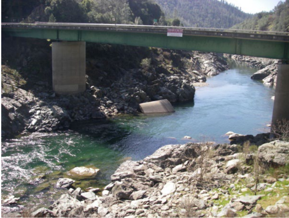
Figure B1.1. Placer-49, PM 0.2. Bridge over North Fork American River.
