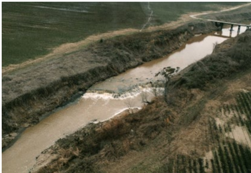
Figure 8. Headcut in Consolidated Cohesive Bed Approaching County Road Bridge
