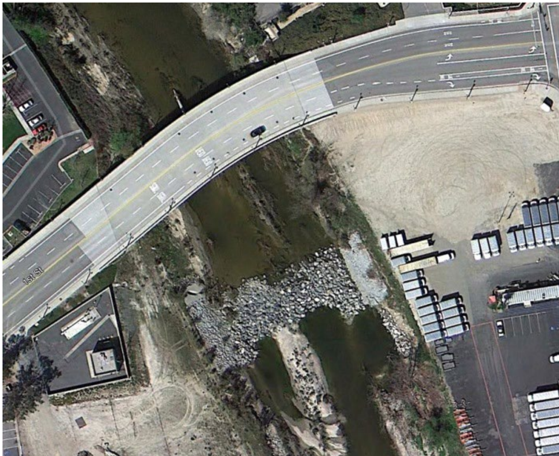
Figure B3.11. Aerial view (2011) of grade control structure constructed downstream from 1st Street Bridge.
