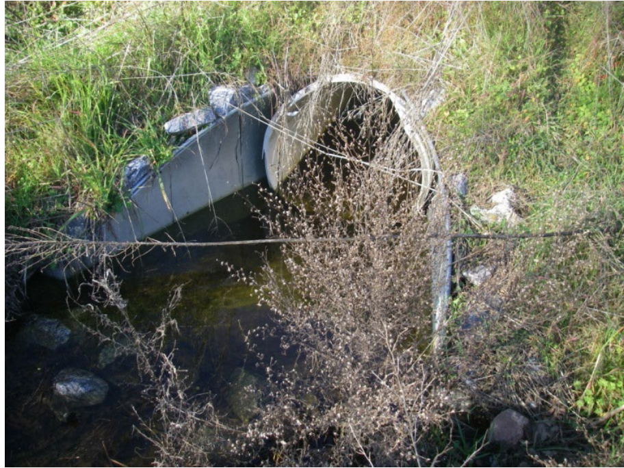
Figure B5.1. Flared outlet for Example 5 culvert.
