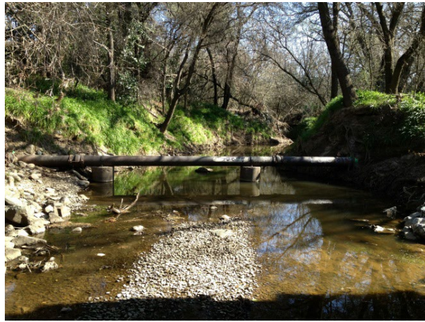
Figure B4.8. Typical Bed Material Size, Arcade Creek site 13. Note exposed pipeline, which is diagnostic of channel incision.
