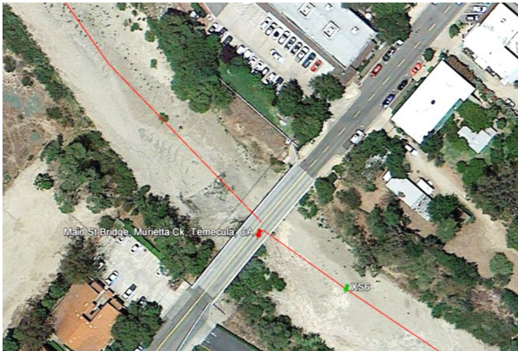
Figure B3.1. Ground level (top) and aerial (bottom) views of Main Street Bridge over Murietta Creek at Temecula, CA.
