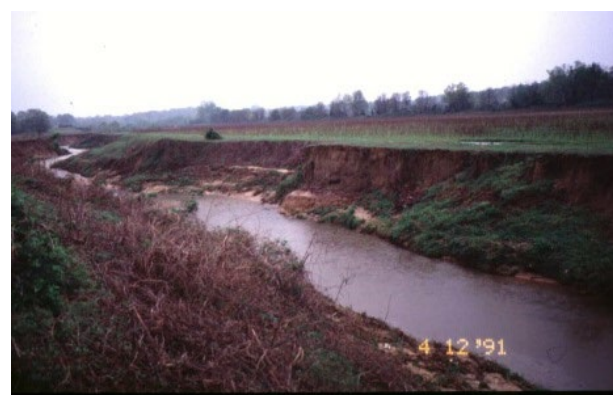
Figure 23. Bank Erosion Examples
