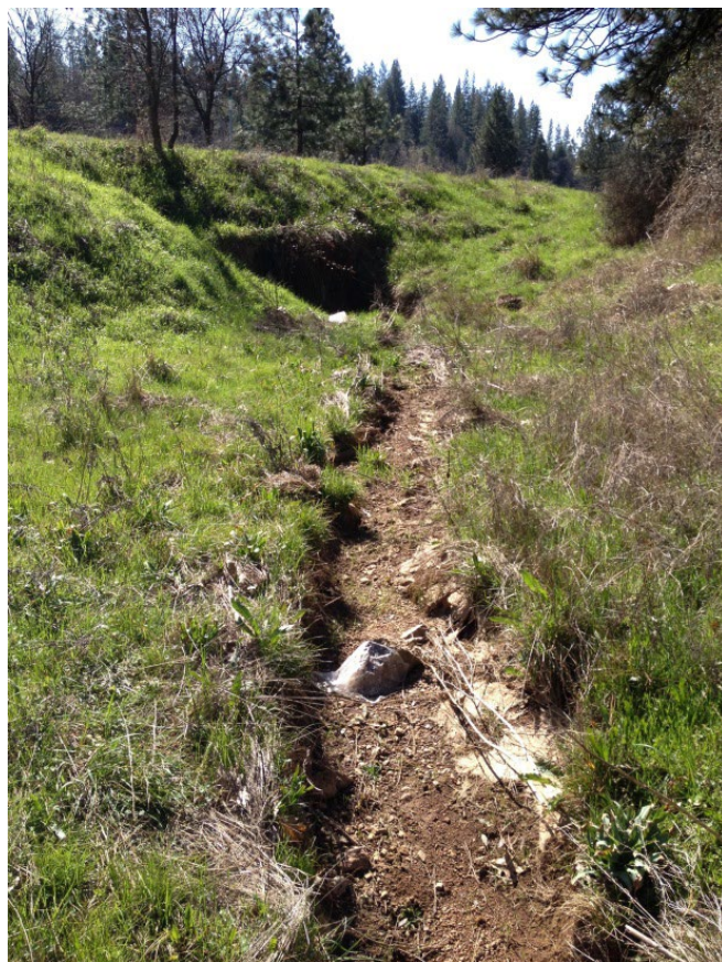
Figure 17. Channel Entrenchment Examples
