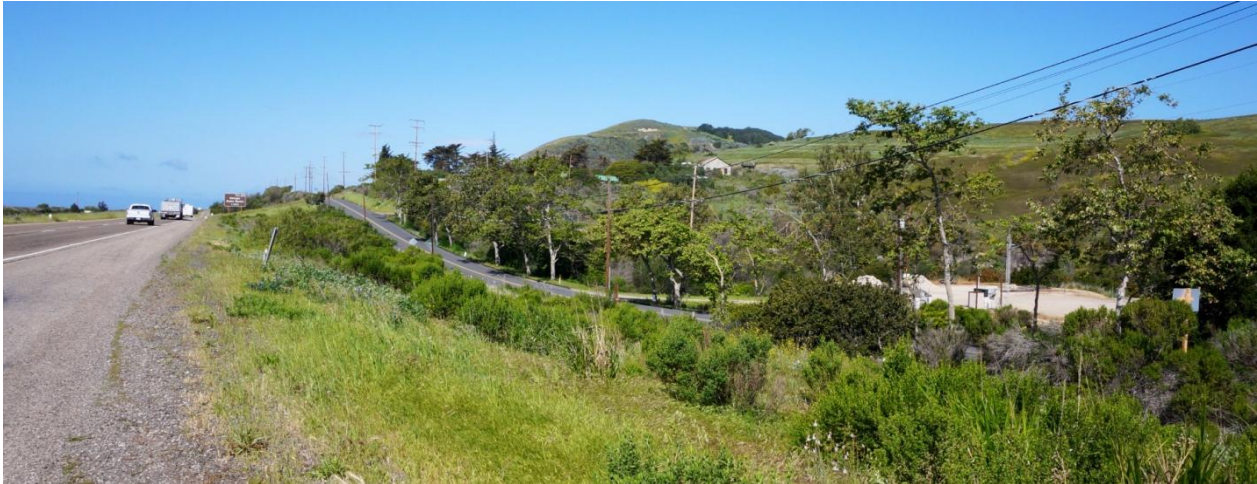
Fig 8.2- Intrusion: Residential homes visible looking north at PM 35.5
