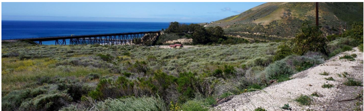
Fig. 22 - Intrusion: A difficult to catch glimpse of Gaviota State Beach looking away from the direction of southbound travel on ocean side of Highway 101 at PM 46.00
