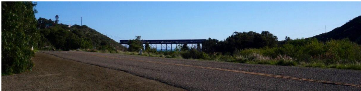
Fig. 21- Intrusion: Historical Railroad trestle visible at PM 46.50
