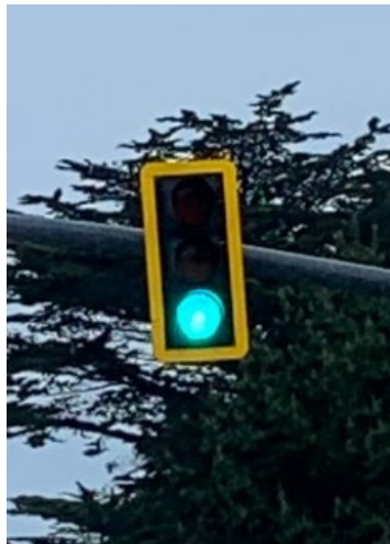
Figure 1 Signal with Retroreflective Border (photo courtesy of Brian Simon)
