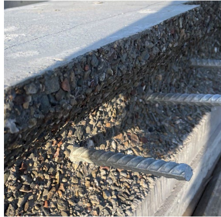
Figure 4.9.5.1.2-2 Longitudinal Keyway with Exposed Aggregate Finish
