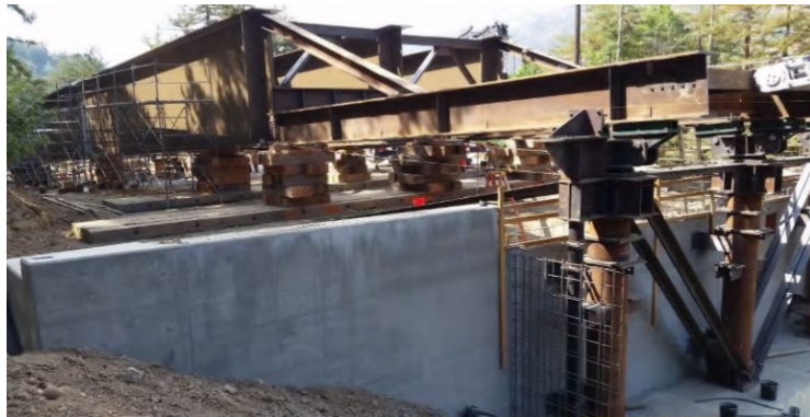
(a) Launch setup at abutment
