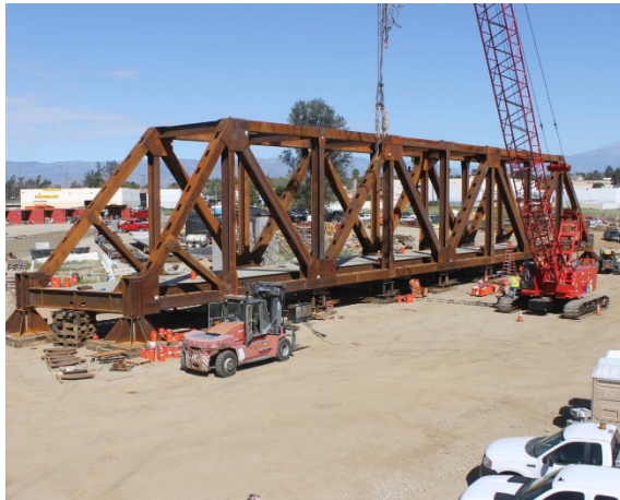
(a) Truss span in the BSA
