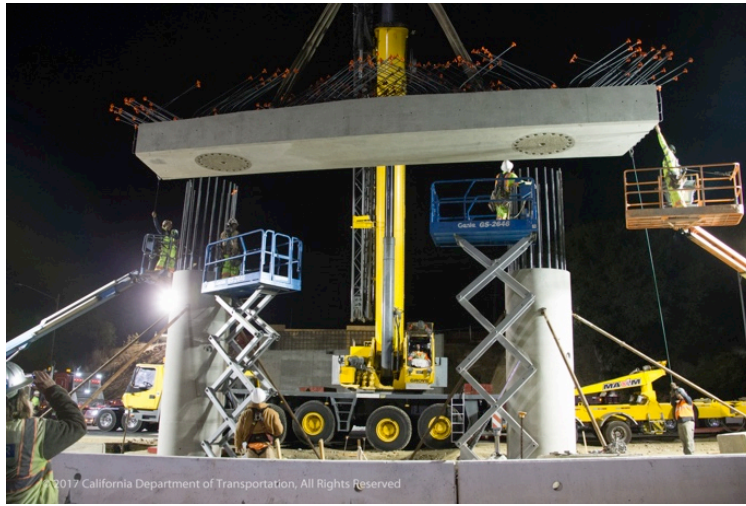
Figure 4.9.4.4.2-1 Laurel Street OC Precast Columns Ready for Bent Cap Assembly
