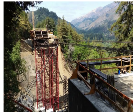
(b) Temporary launch tower
