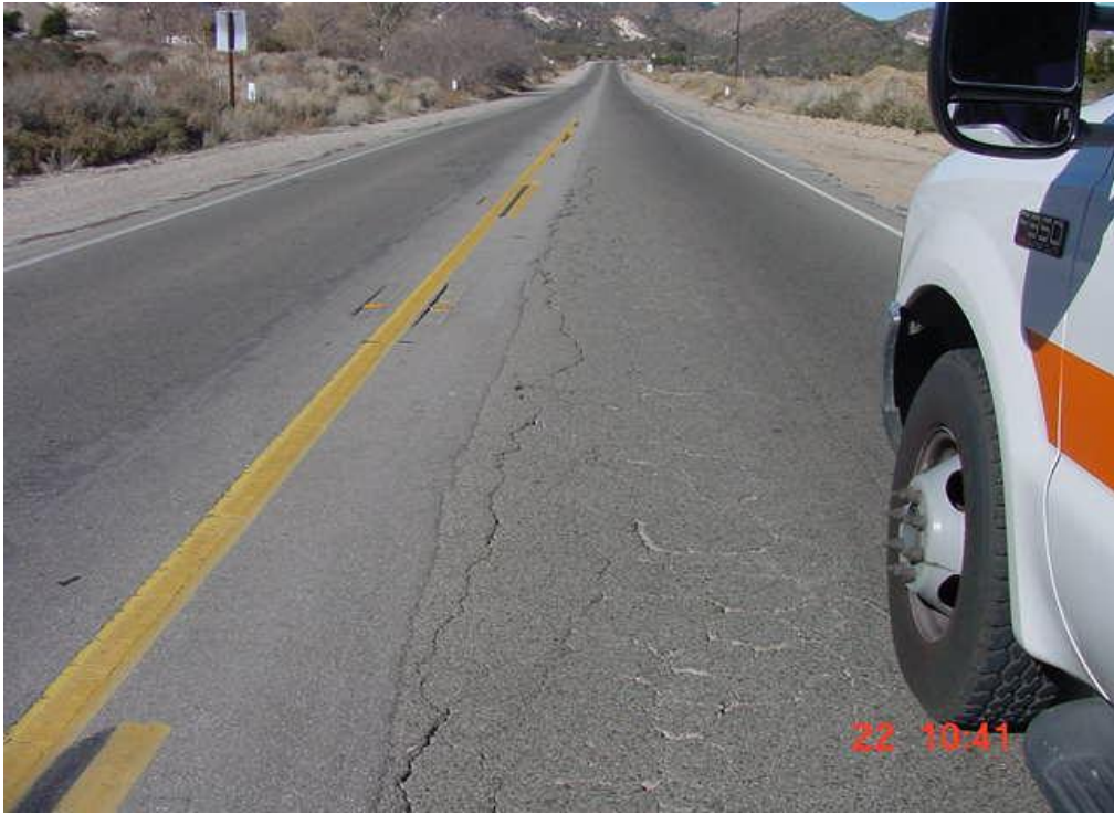
FIGURE 5. An Example Photograph of a Test Section
