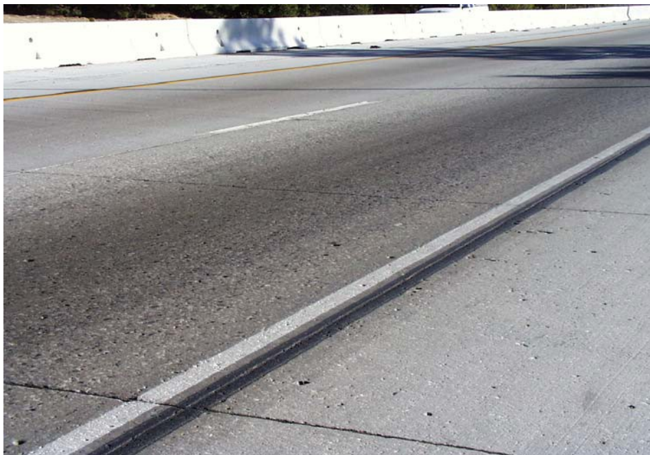
Photo 2: Black contrast stripes can increase the conspicuity of traffic striping on light-colored PCC pavements, especially in areas with PCC shoulders.
