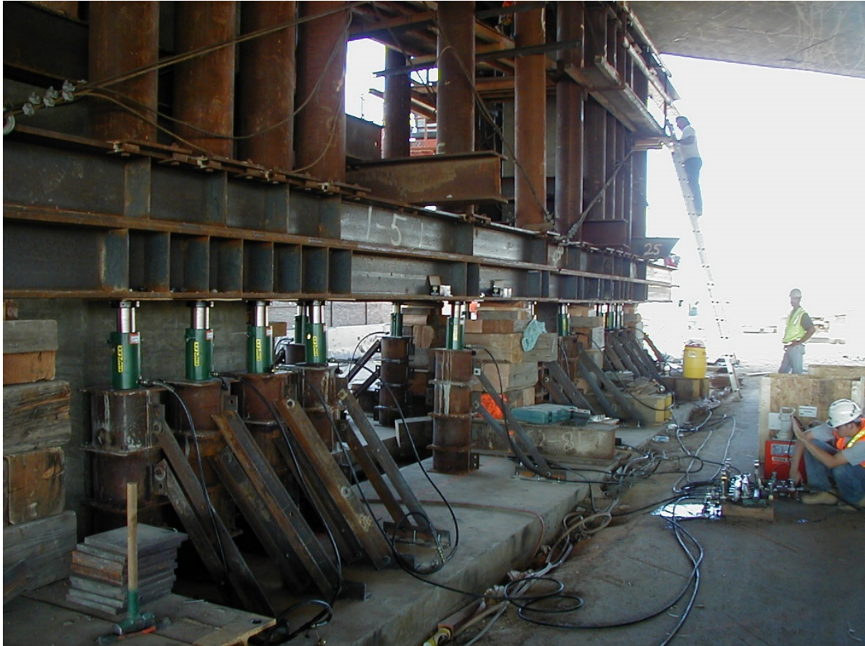
Figure 1. A fairly typical jacking system. Note the restraint of the cap beam to prevent unwanted movement.
