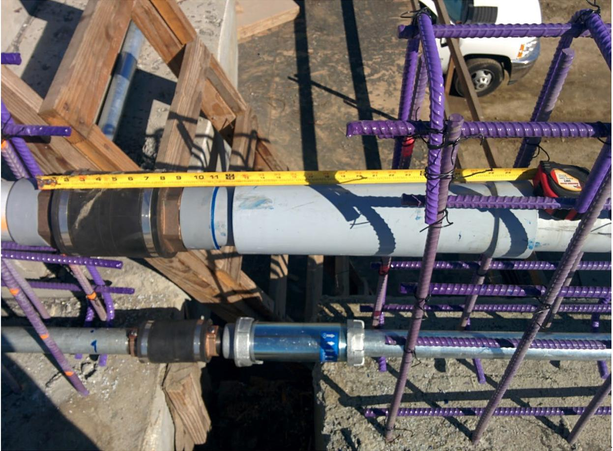
**Figure 6. Conduit Expansion Coupler at Bridge or Wall Joint**
