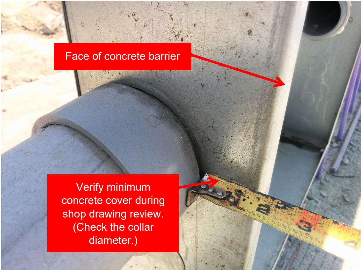
**Figure 5. Check Anticipated Concrete Cover over Rebar and Conduit**
