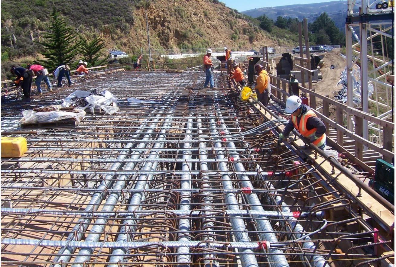
**Figure 4. Transverse Prestressing Ducts and Tendons in Bridge Deck**
