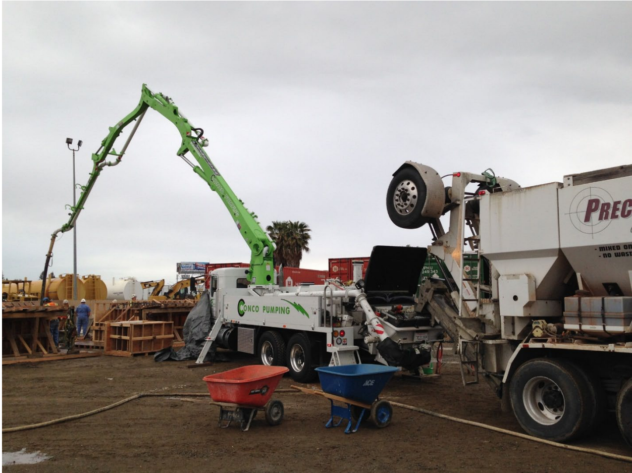
Figure 4. Volumetric mixer staging with pump truck pumping into a mock-up
