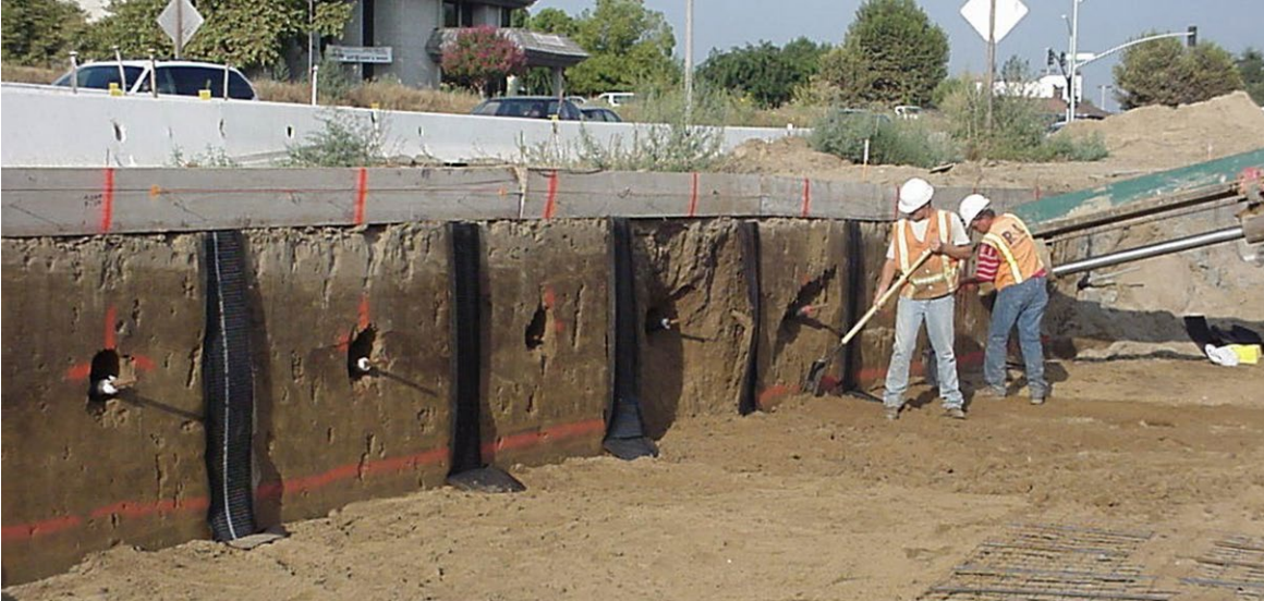
Figure 3. Material that stands initially, may slough over time as the soil loses moisture. Thus, even apparently good soil material may slough.
