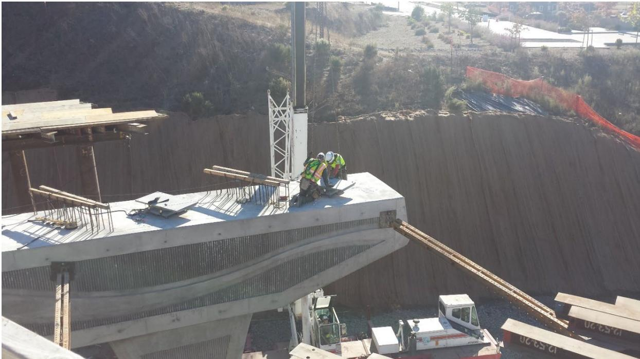
**Figure 3. Installation of PTFE Spherical Bearings (Petaluma River Bridge Project)**
