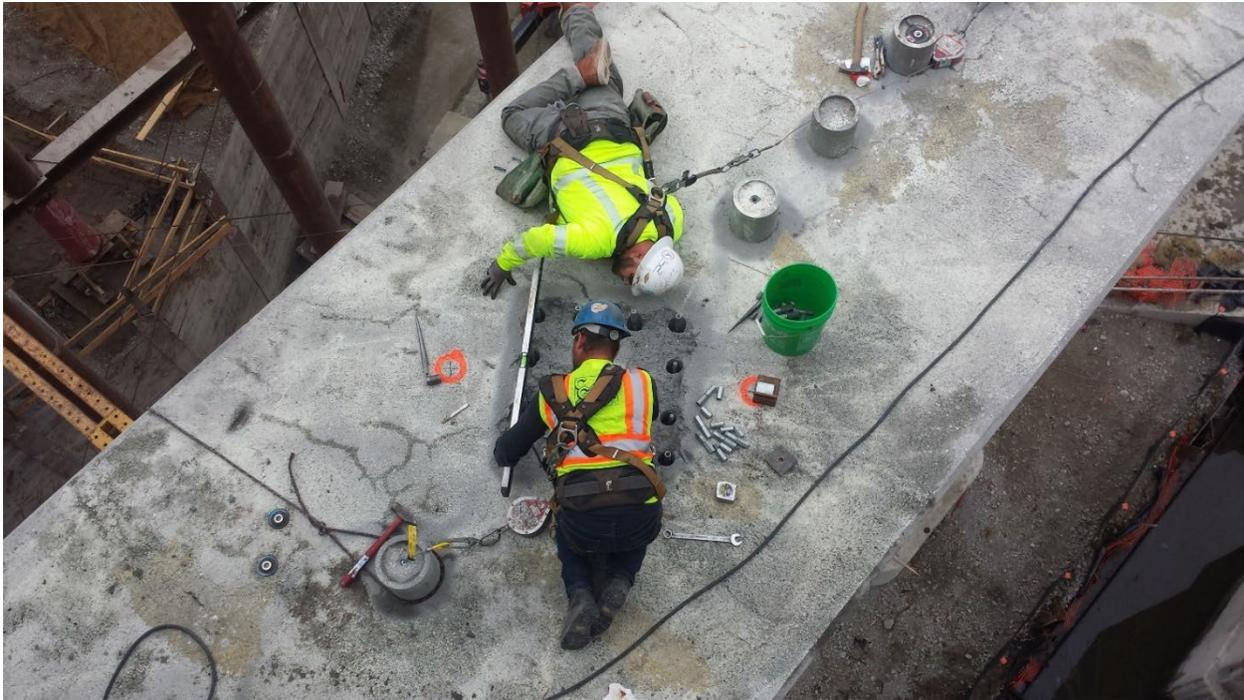
**Figure 2. Lug Installation and Checking the Level of the Concrete Surface to Receive the PTFE Spherical Bearing (Petaluma River Bridge Project)**
