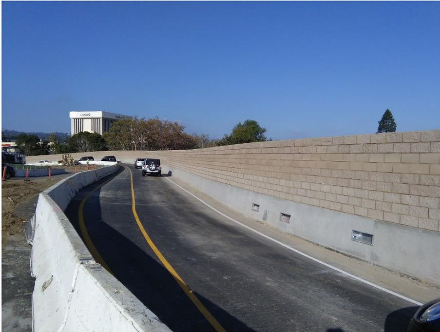
**Figure 1. Masonry Block Sound Wall in San Mateo, CA on Hwy 92, EA 04-235524**
