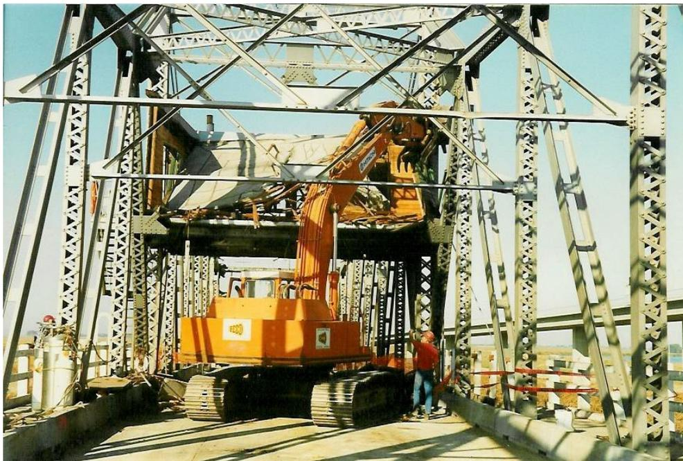
**Figure 3-3. Excavator Removing Control House, Potato Slough**
