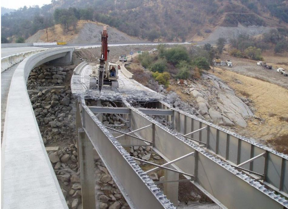
Figure 3-4. Excavator Removing Concrete Deck on Steel Girders
