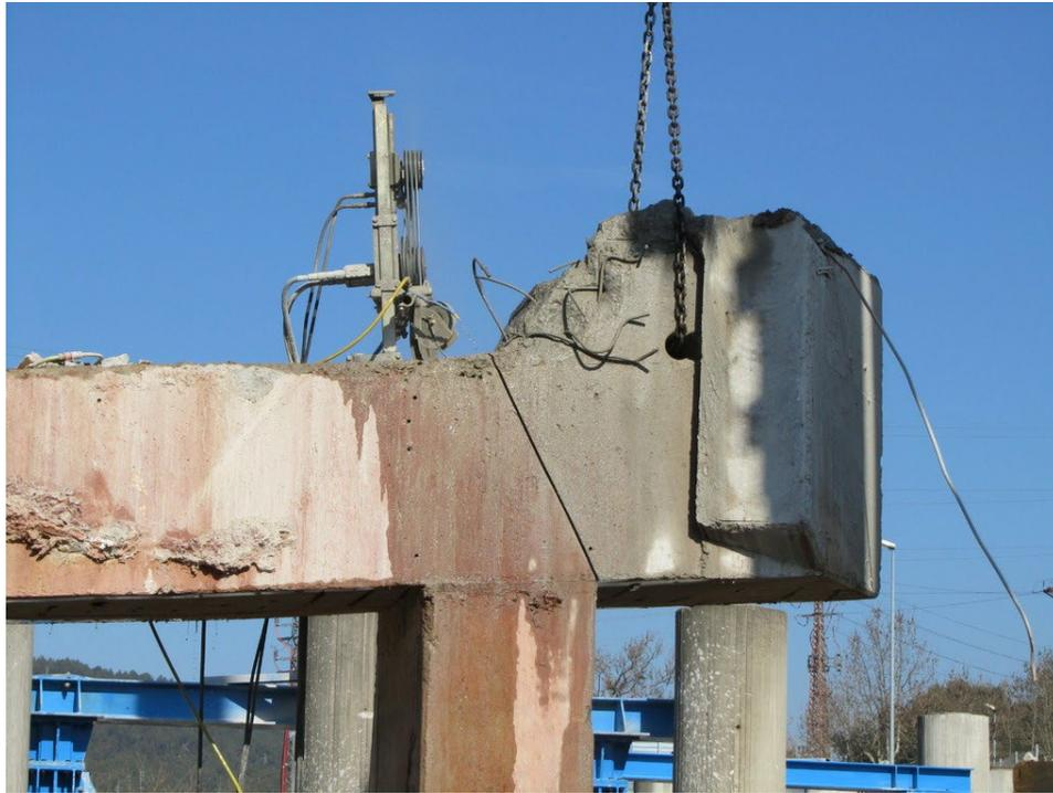
Figure 3-7. Diamond Wire Saw
