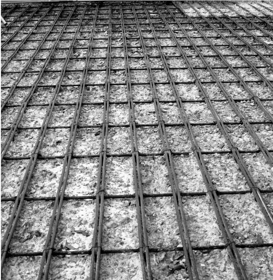
Figure 3-12. Hydroblasting for Partial Deck Removal
