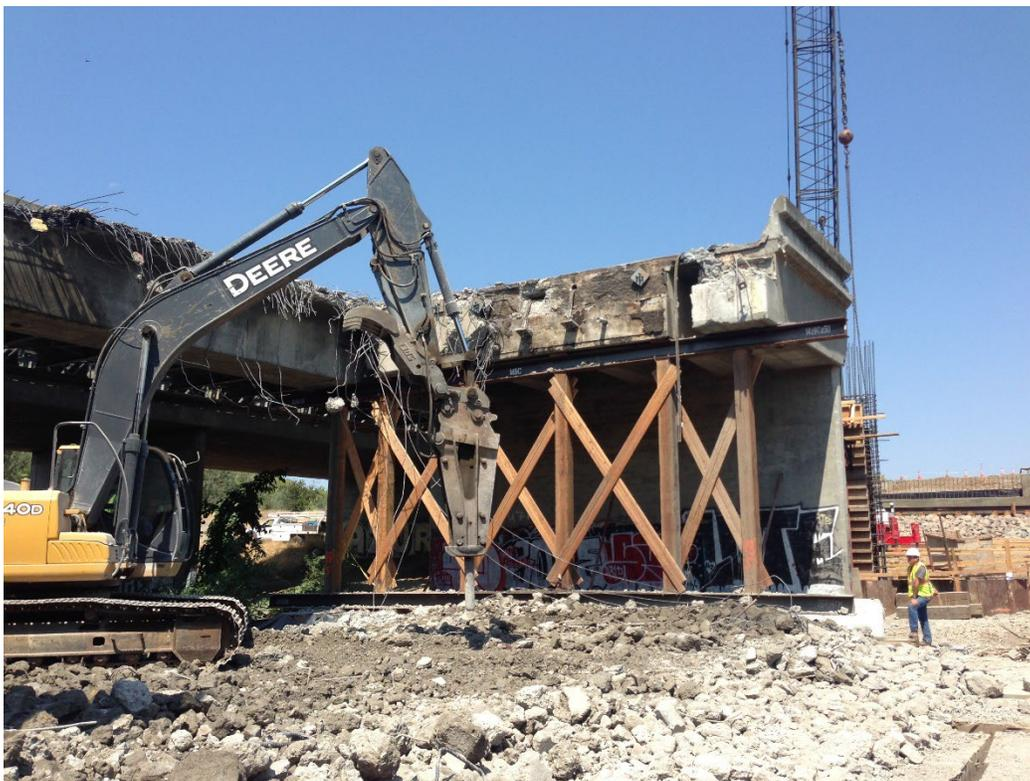
**Figure 3-15. Temporary Support for Bridge Removal, Chico**
