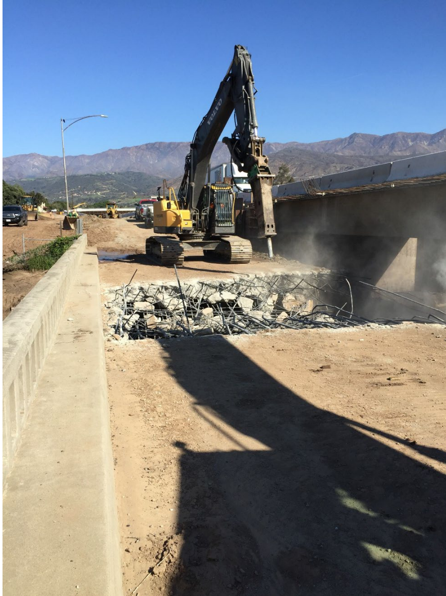
Figure 4-2. Typical Equipment Live Load, Carpinteria Creek
