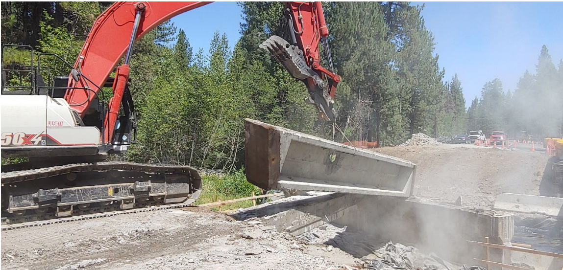
Figure 4-4. Precast Girder Removal with Excavator, Hat Creek
