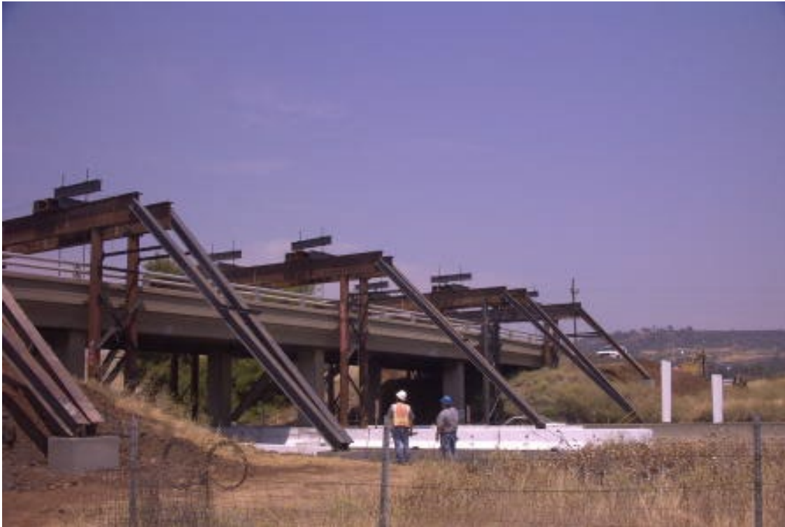
Figure 4-3. Temporary Support During Partial Removal and Bridge Raising, Oroville
