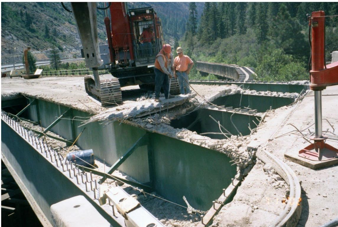
**Figure 6-12. Bridge Deck Removal from Steel Girders, Acid Flat**
