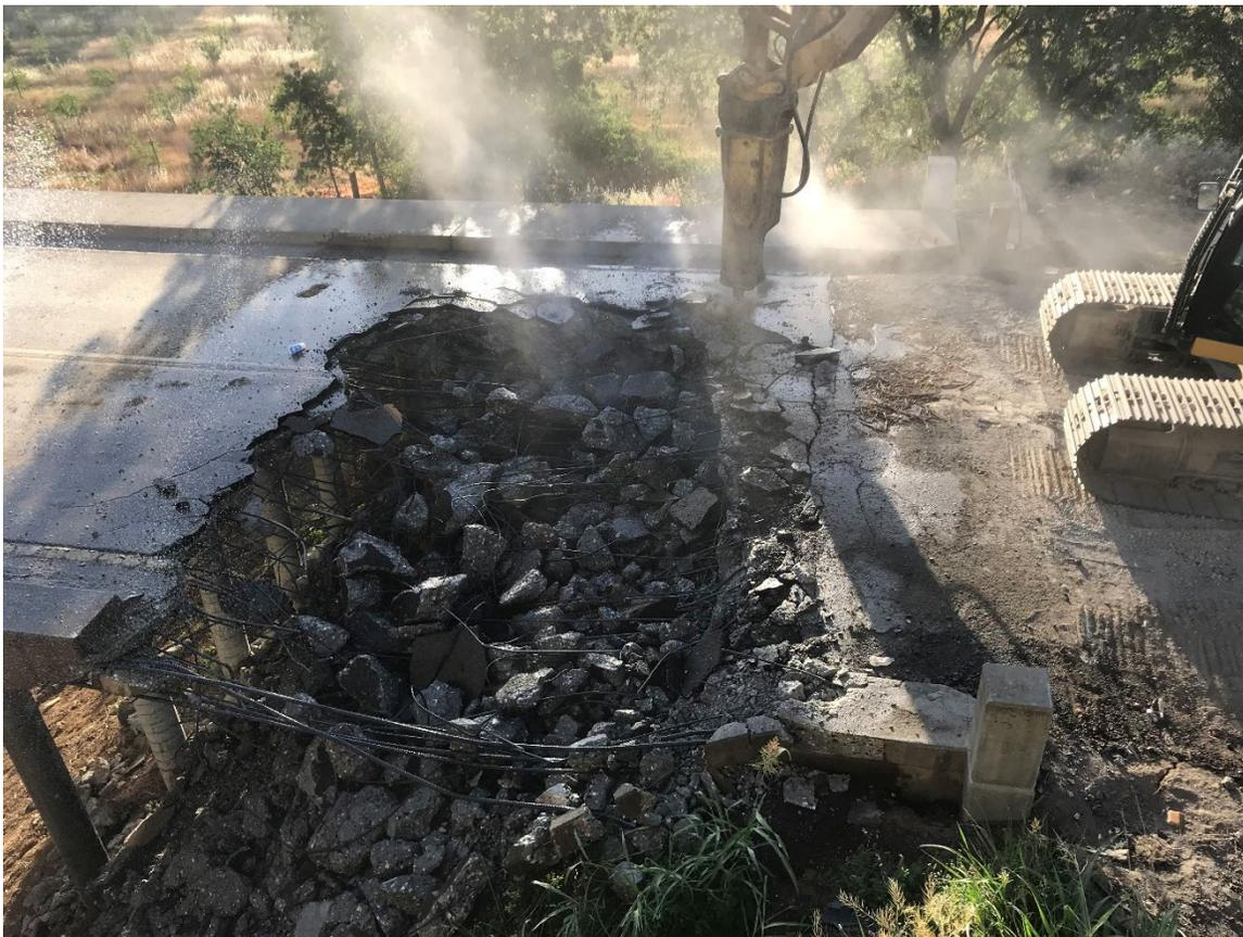
**Figure 6-11. Slab Deck Removal, Simmerly Slough**
