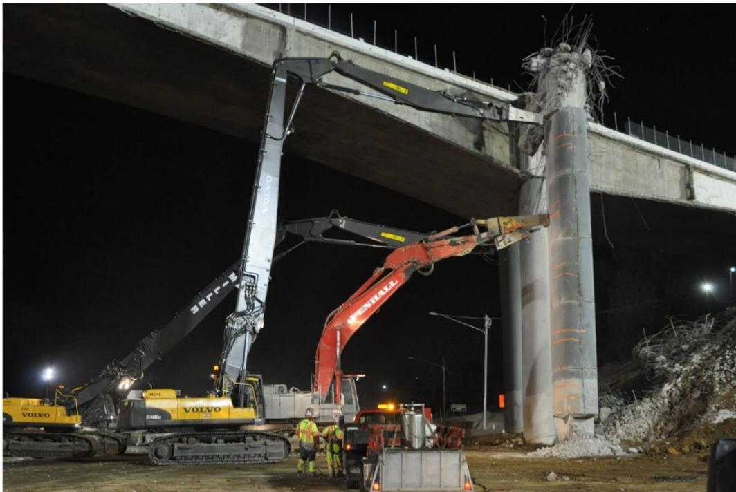
**Figure 6-22. Column Removal by Pushover after Weakening Base, Mulholland Drive, Los Angeles**
