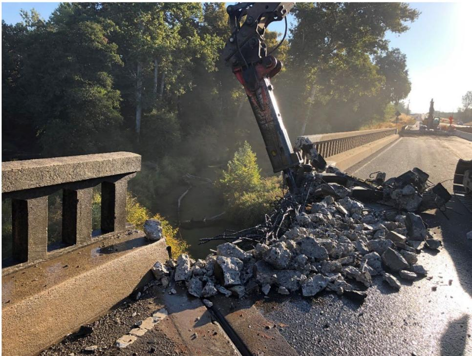
**Figure 6-7. Barrier Rail Removal, Dry Creek**
