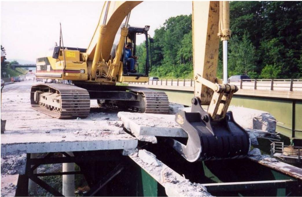
**Figure 6-9. Slab Removal Attachment on Excavator**
