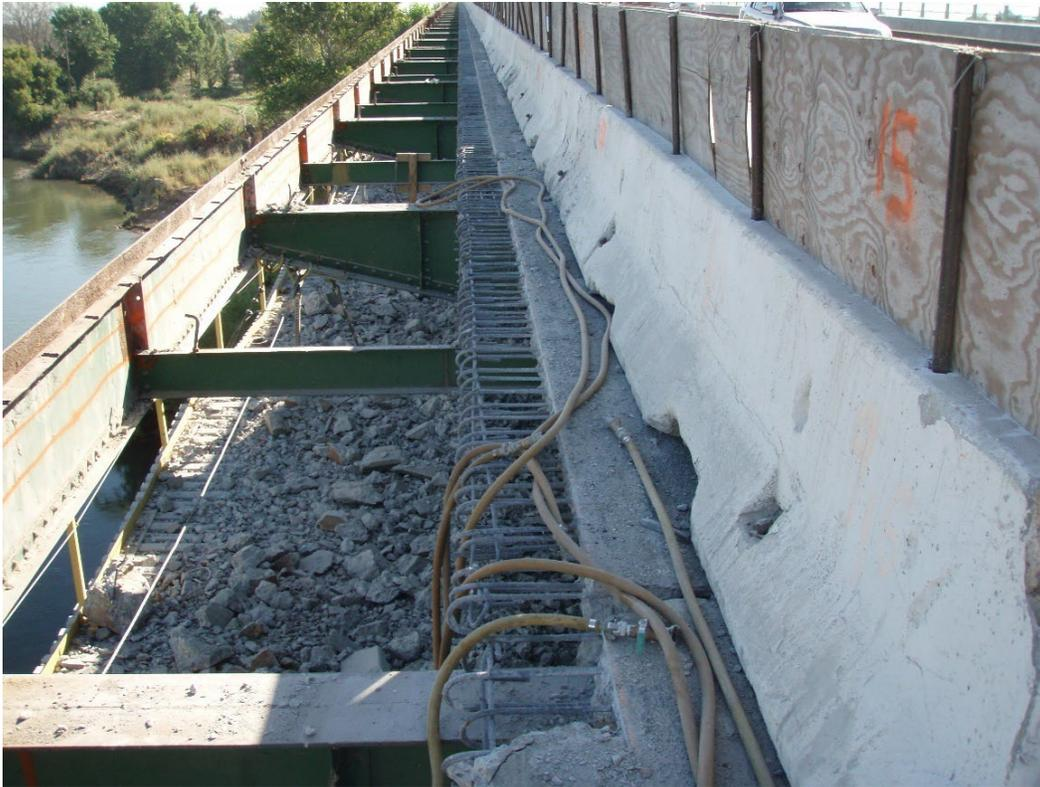
**Figure 6-6. Suspended Debris Containment Platform**
