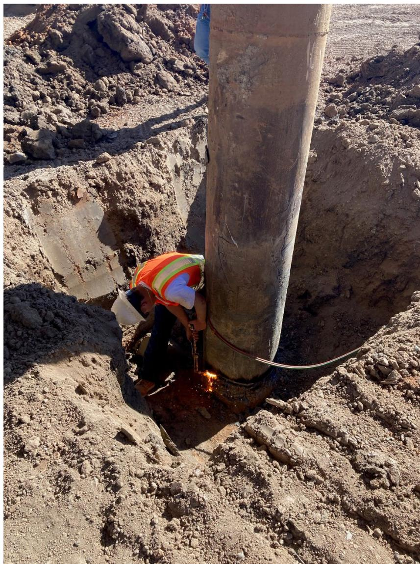
Figure 6-27. Piling Removal Below Grade, Simmerly Slough
