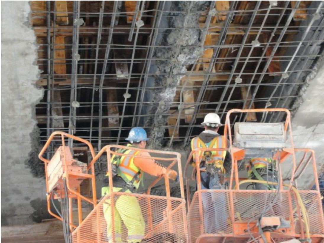
Figure 8-4. Soffit Repair at Doyle Drive, San Francisco
