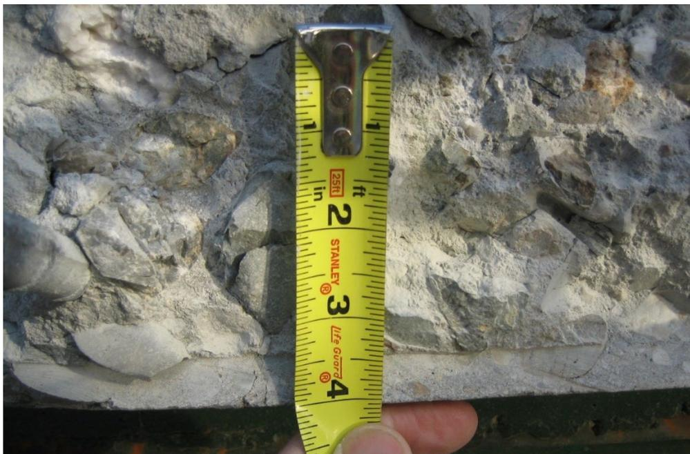
Figure 8-1. An Inspector Documents the Depth of Soffit Saw Cut
