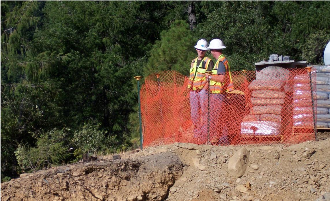
Figure 7-9. High Visibility Fencing used for ESAs
