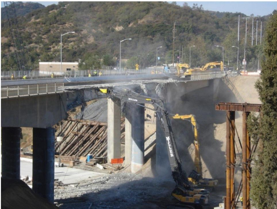
Figure 3-1. Long Reach Excavator at Mulholland Drive, Los Angeles
