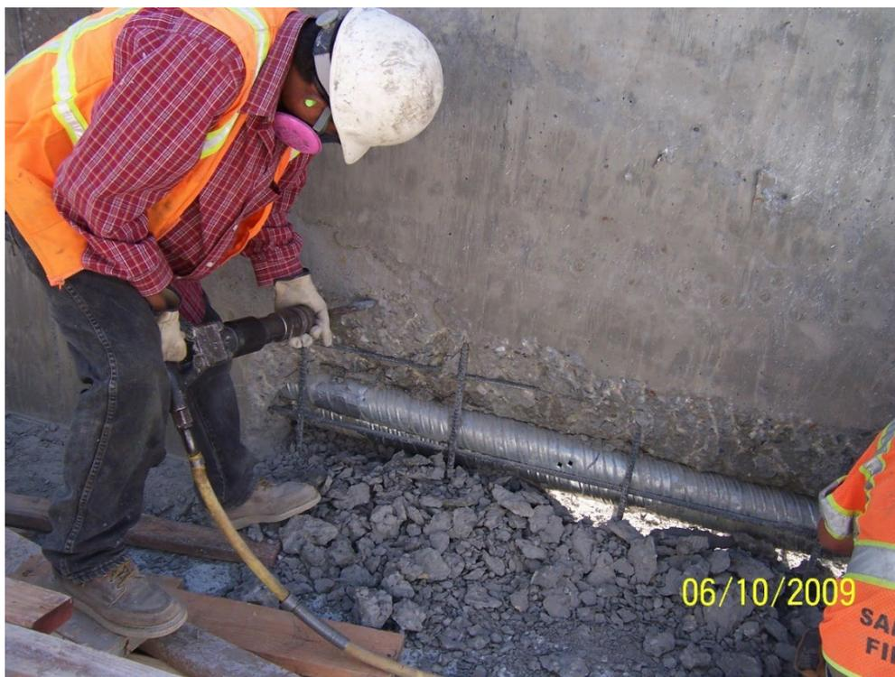
Figure 3-9. Handheld Pneumatic Hammer, Bear River
