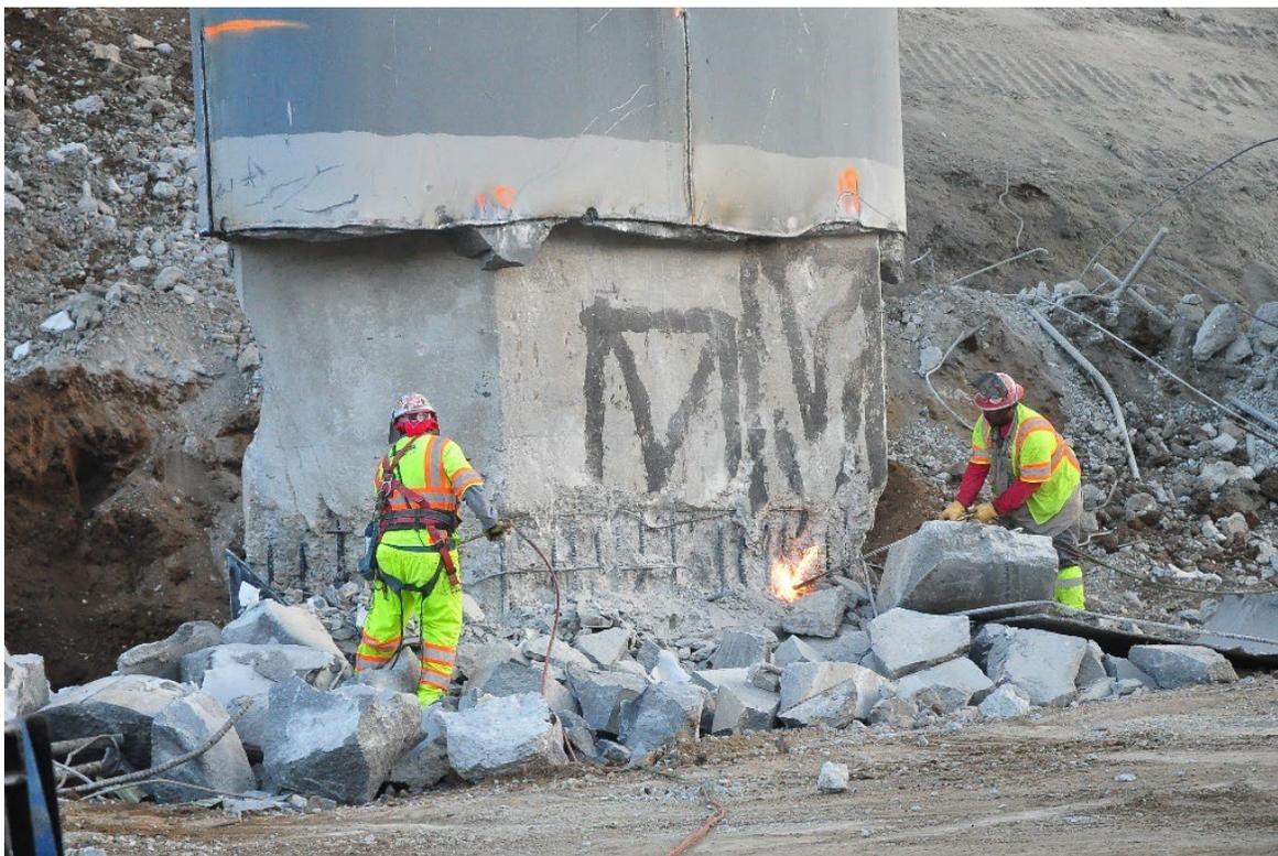
Figure 3-11. Torches Removing Column Reinforcement, Mulholland Drive, Los Angeles
