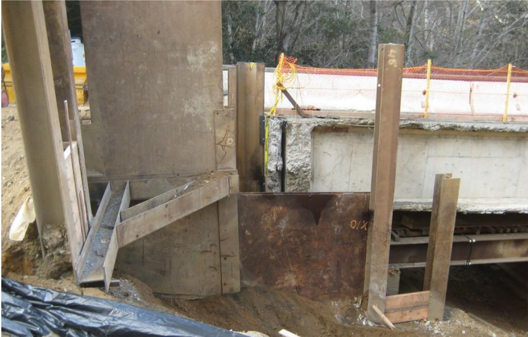
Figure 6-25. Partial Abutment Removal with Shoring and Temporary Support, Greenwood Creek
