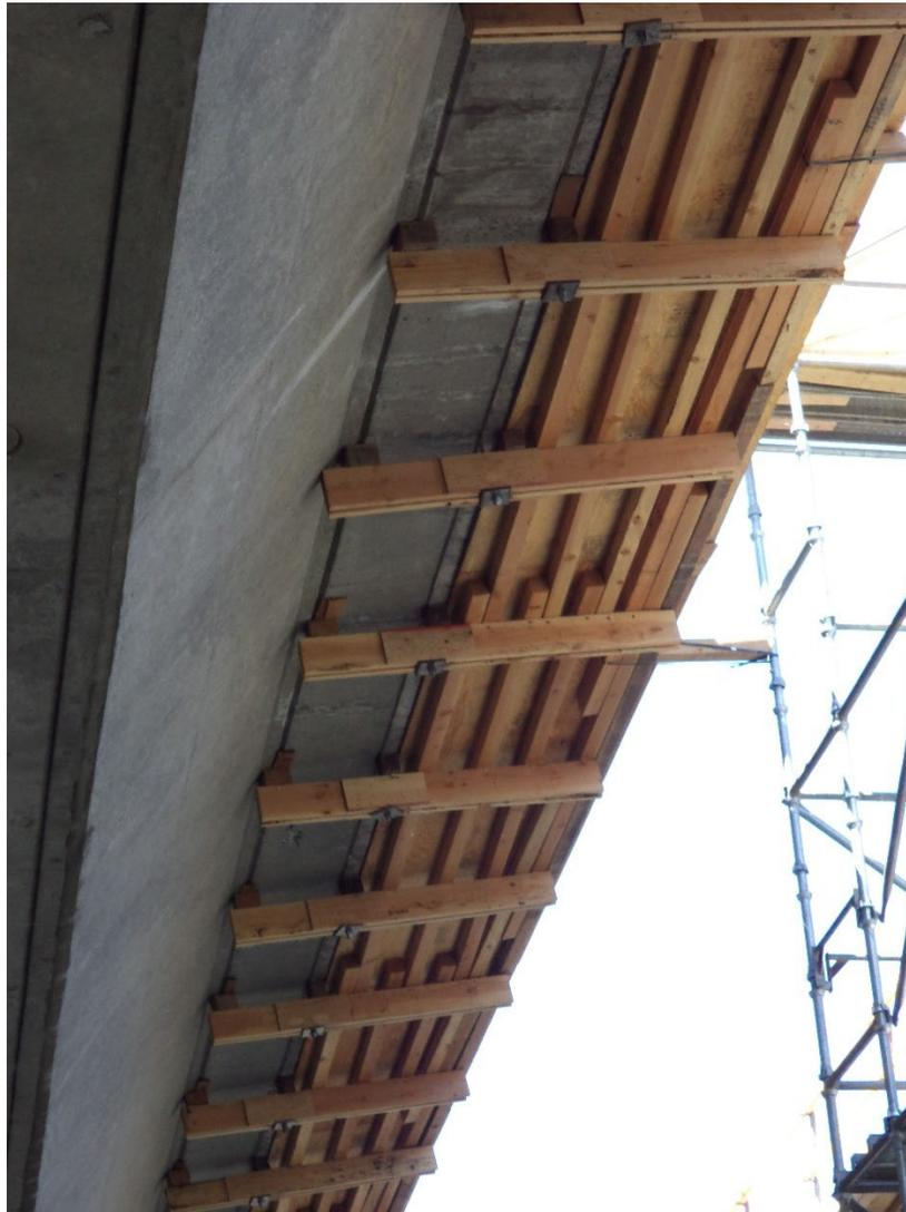
**Figure 5-5. Four-Foot-Wide Protective Cover for Rail Removal, Sacramento**
