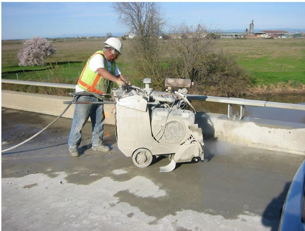
Figure 3-6. Water Cooled Concrete Saw
