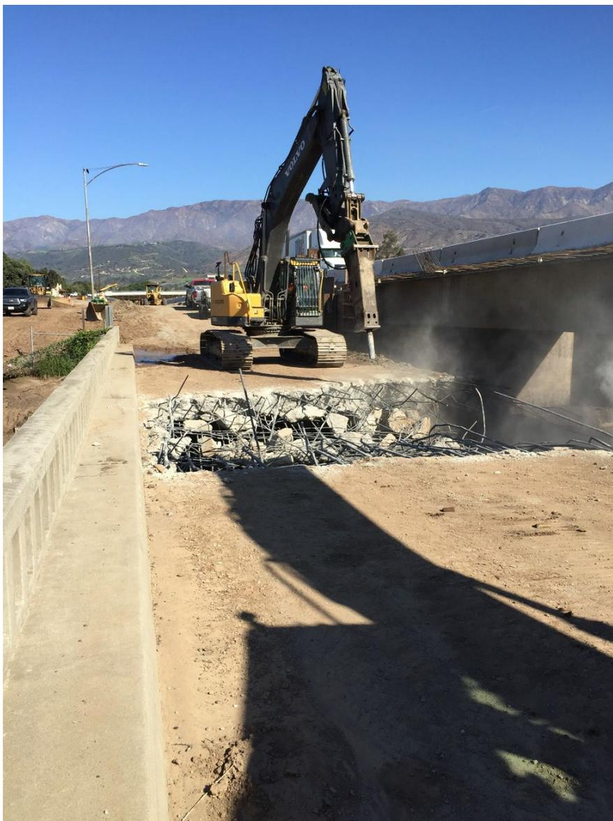
Figure 4-2. Typical Equipment Live Load, Carpinteria Creek
