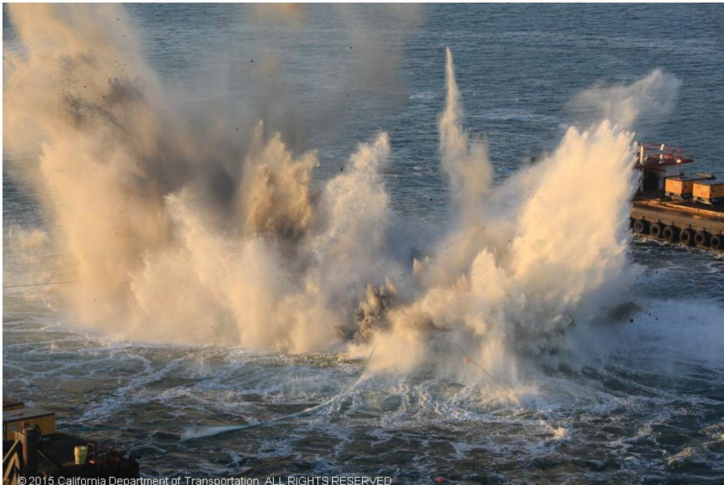
Figure 3-14. Explosive Demolition of a San Francisco-Oakland Bay Bridge Pier
