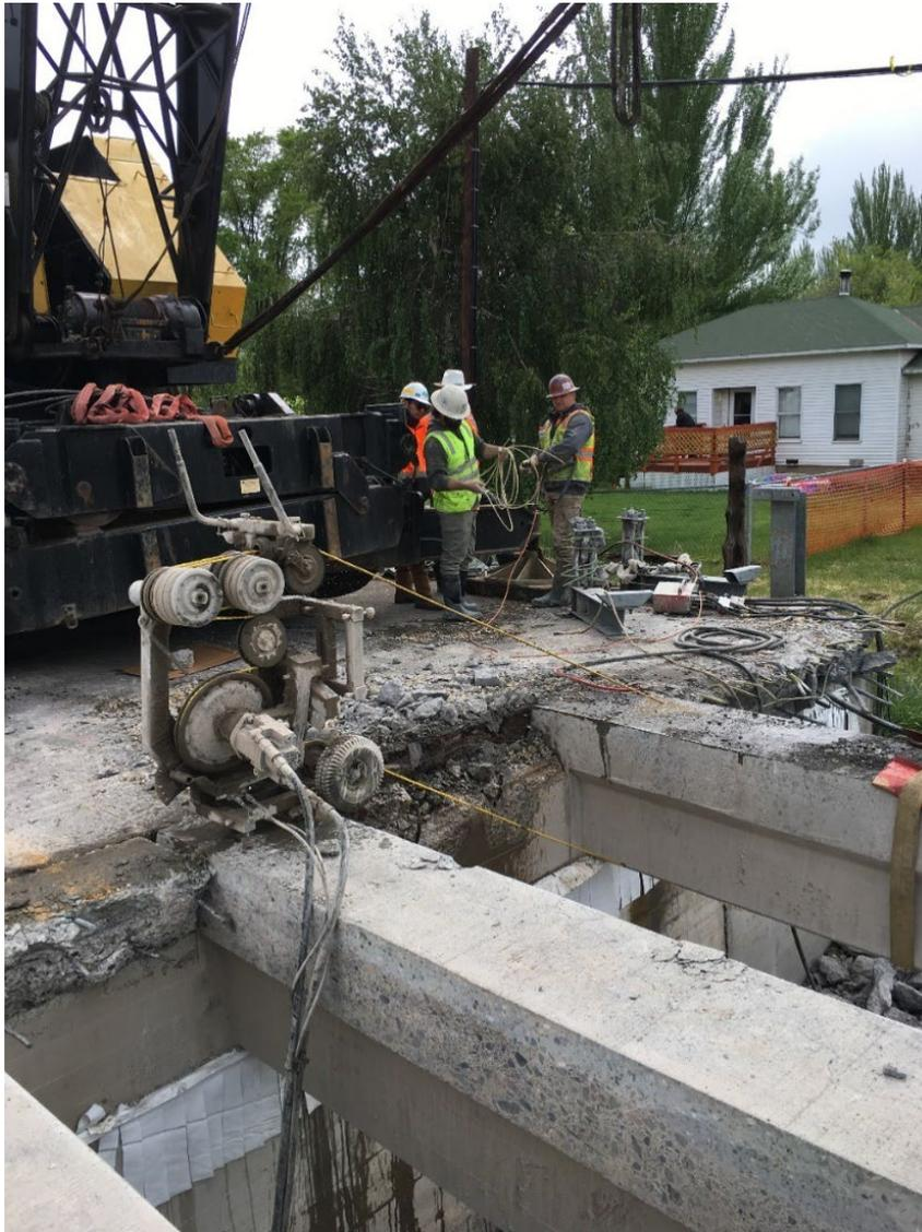
Figure 6-19. Wire Saw Cutting Concrete Girder Supported by a Crane
