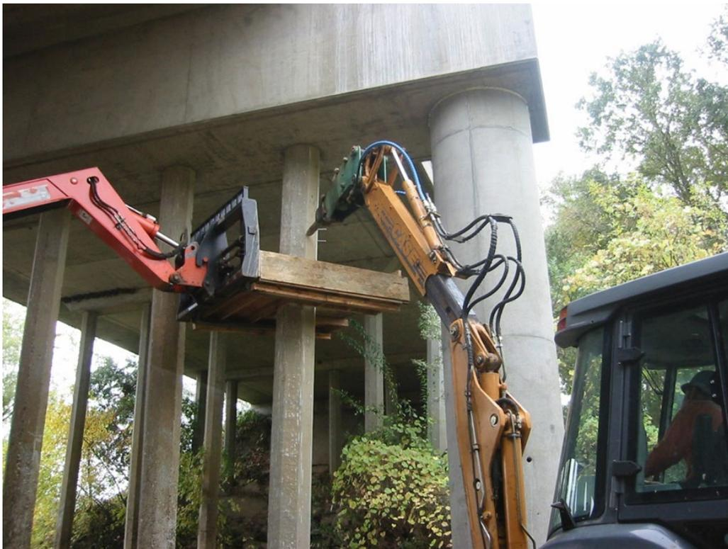
**Figure 7-2. Debris Containment Platform, Honcut Creek**
