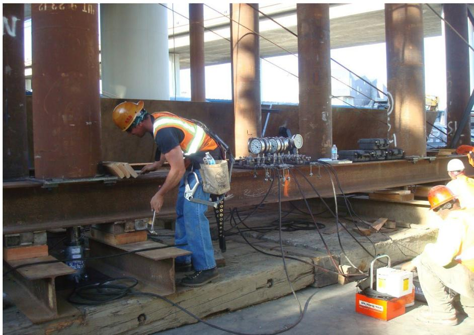
Figure 3-19. Jacking System Transferring Load to Temporary Support, San Francisco
