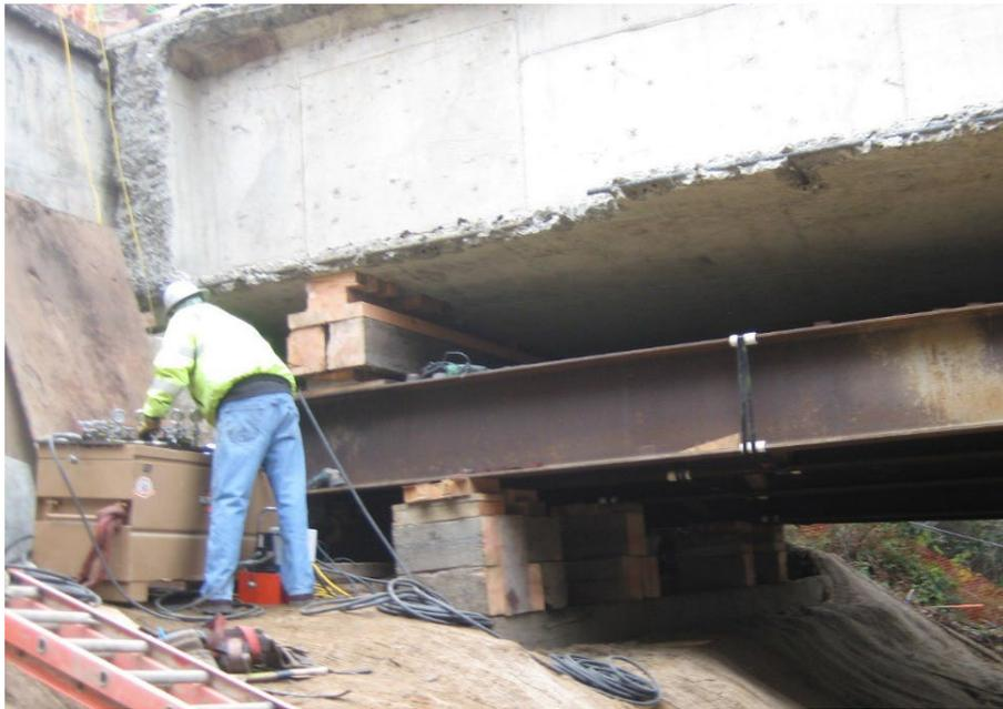
**Figure 3-17. Combined Temporary Supports, Falsework, and Protective Cover, Elk**
