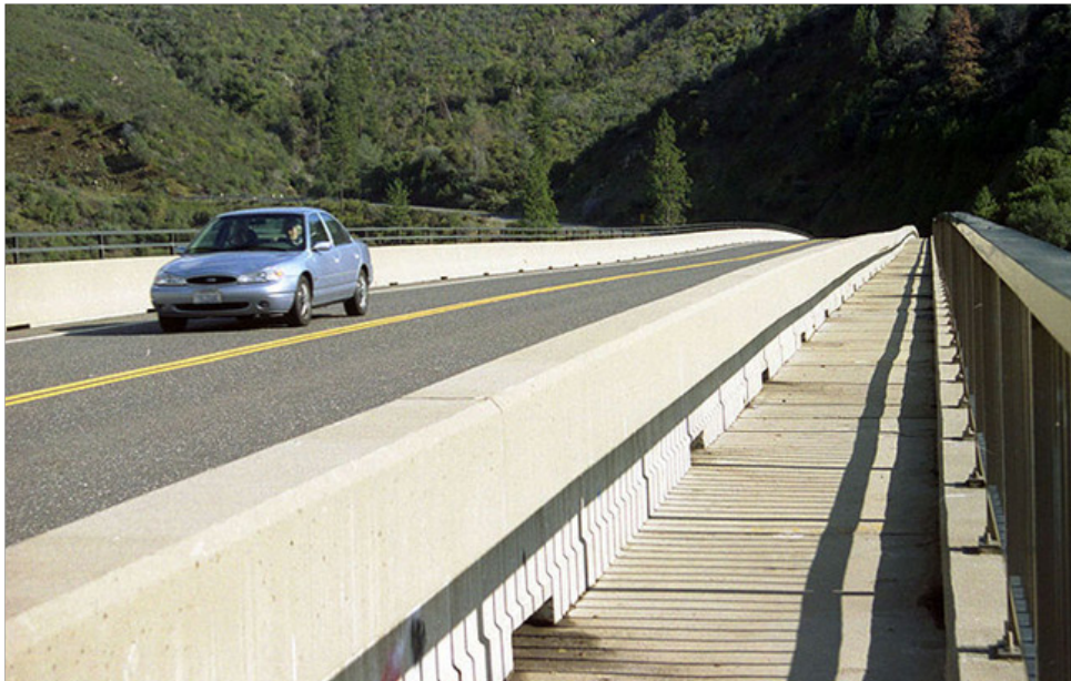
Figure 1-3. Parrotts Ferry Bridge, New Melones River, 22 Inch-Deflection 2 .
