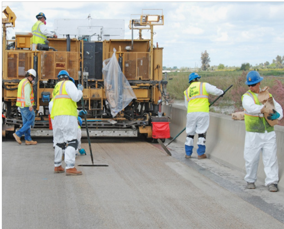
Figure 6-18. Laser Guided Screed.
