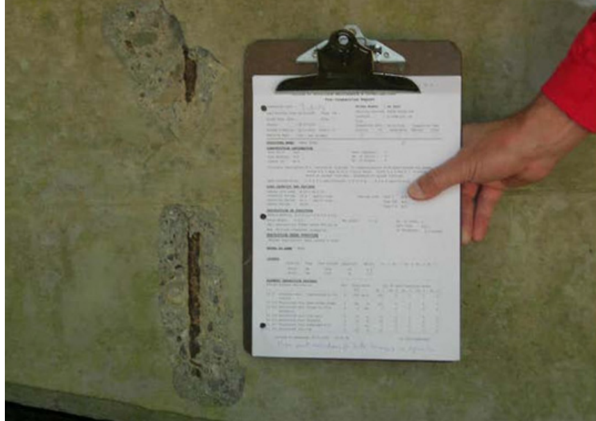
Figure 6-5. Spalling
