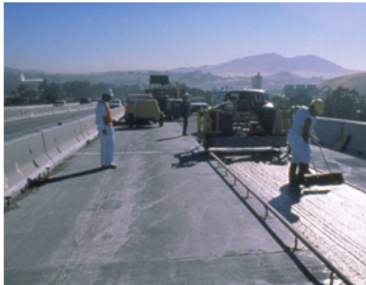
Figure 6-20. Rail Grade Control.
