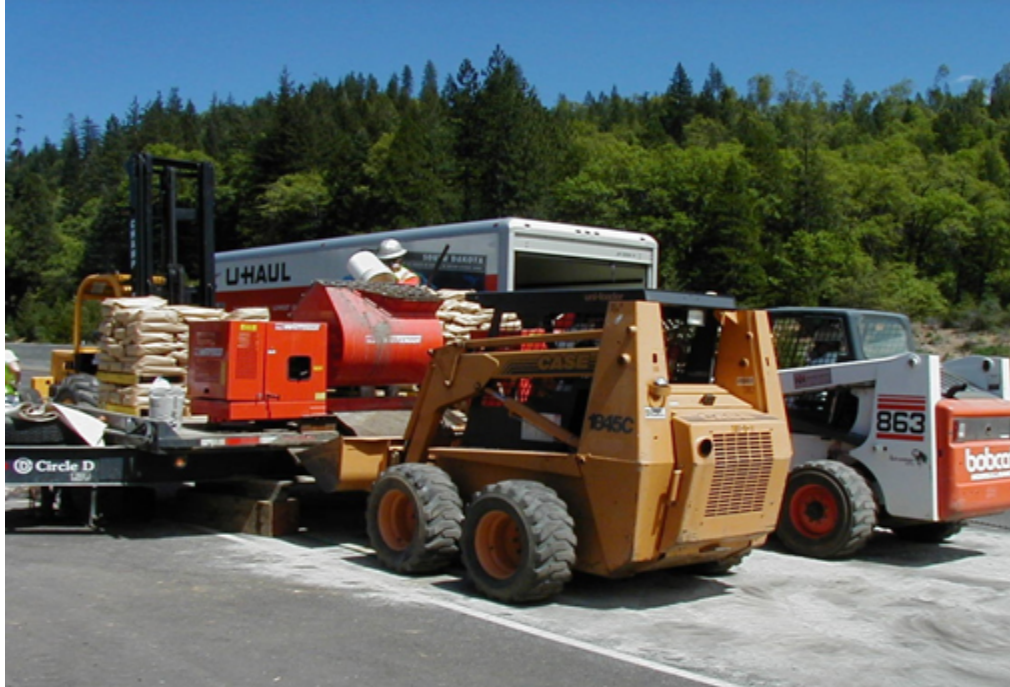
Figure 6-15. Mobile Mixer Operation.
