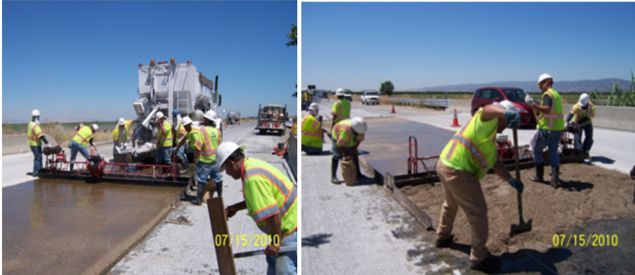
Figure 6-17. “Texas” Screed with Ski Controlled Grading.
