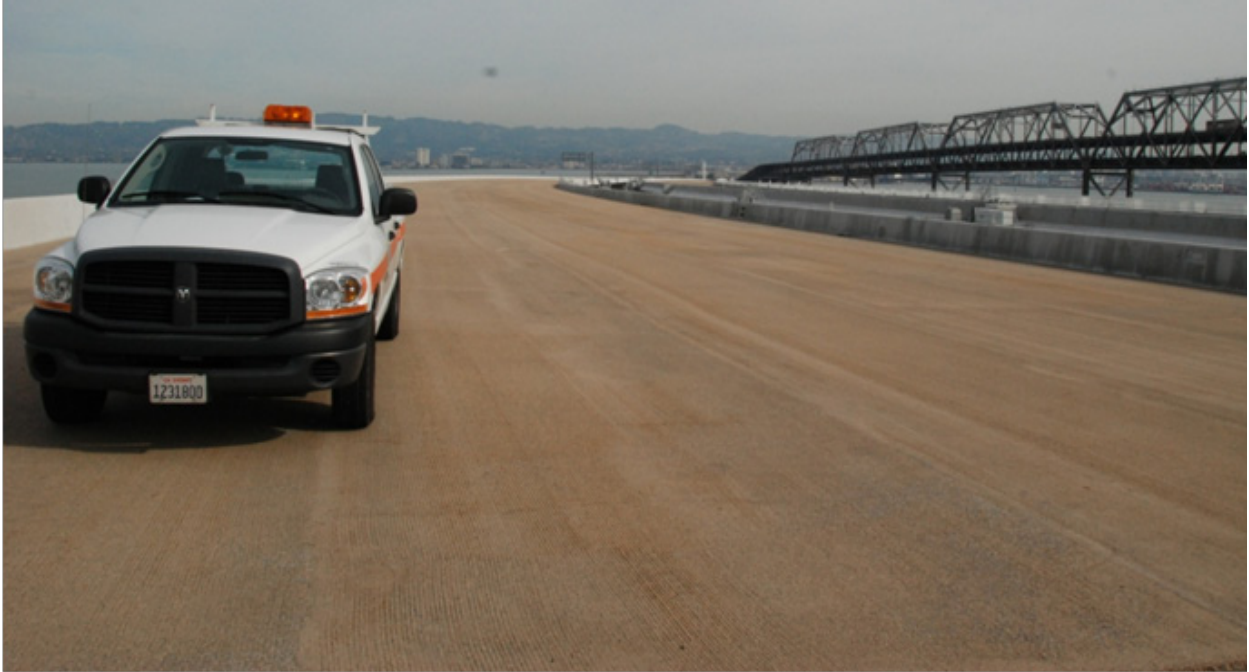
Figure 6-14. Newly Applied Polyester Concrete Overlay.
