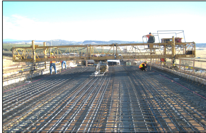
Figure 4.2-4. Inspect Adjustment of the Finishing Machine.
