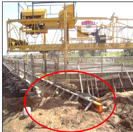
Figure 4.2-2. Screed Rail Should Extend Beyond Pour Area.
