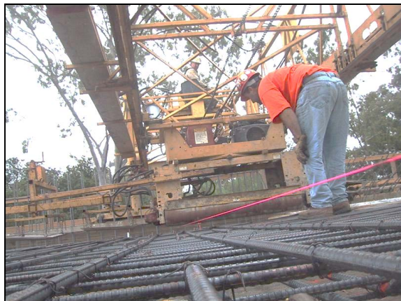
Figure 4.2-5. Check Finishing Machine Height.
