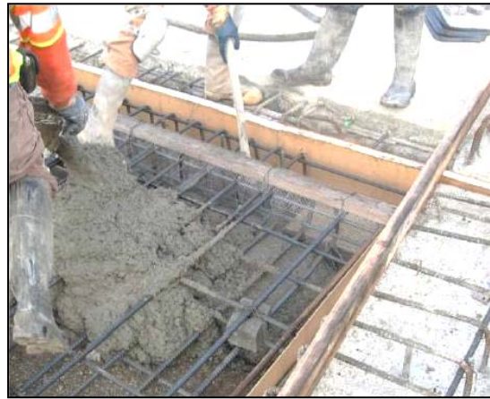
Figure 4.2-3. Check Carefully to Avoid Creating a Bump.
