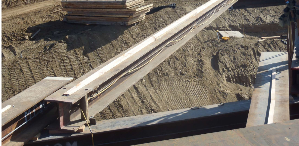
Figure 4-1. Sleeper on the Falsework Stringer
