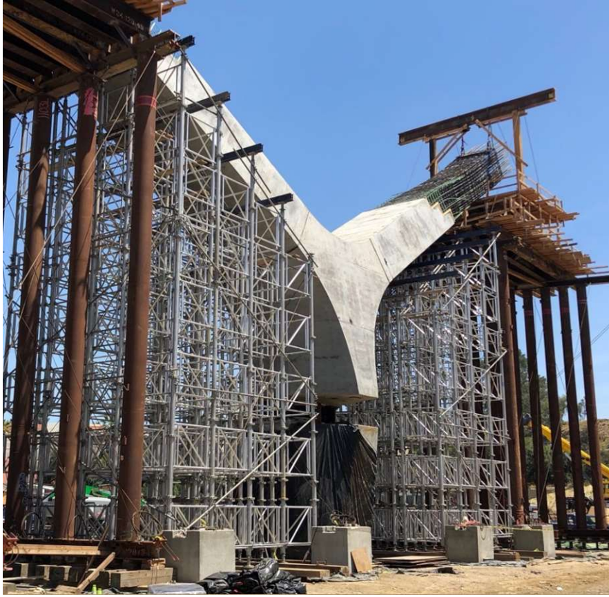
Figure 7-13. Heavy Duty Shoring System.
