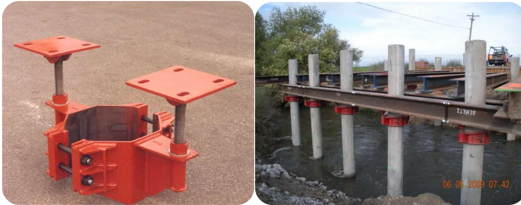
Figure 7-11. Pile Friction Collar.
