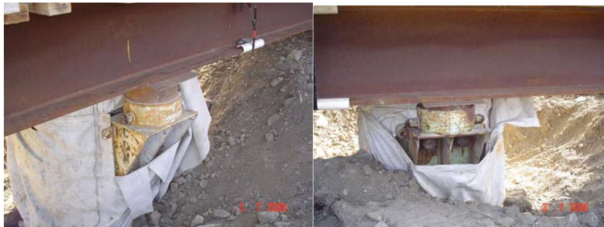
Figure 9-2. Steel Sand Jacks.
