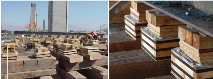
Figure 9-1. Wood Sand Jacks.
