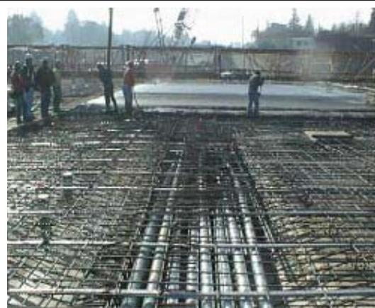
Photo 3-6 – Transverse and Longitudinal Ducts
