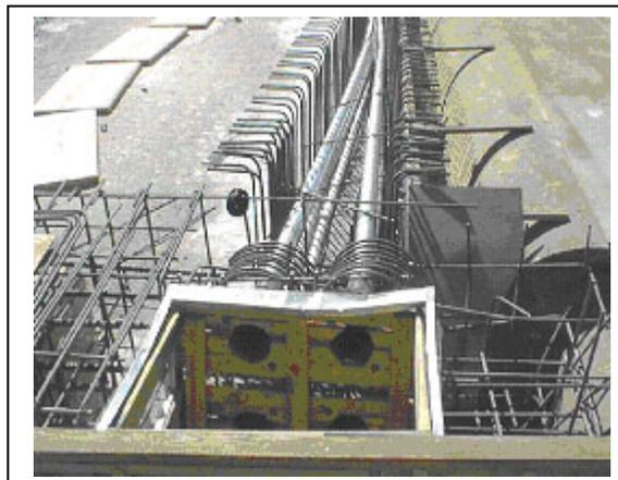
**Photo 5-2 – Blockout for Anchorage Devices.**
