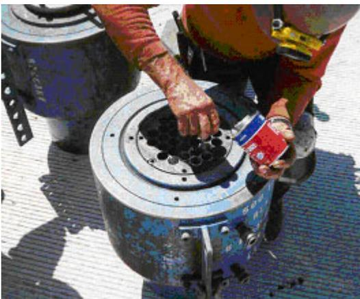
**Photo 6-1 – Pulling Wedges Inserted into Jack**
