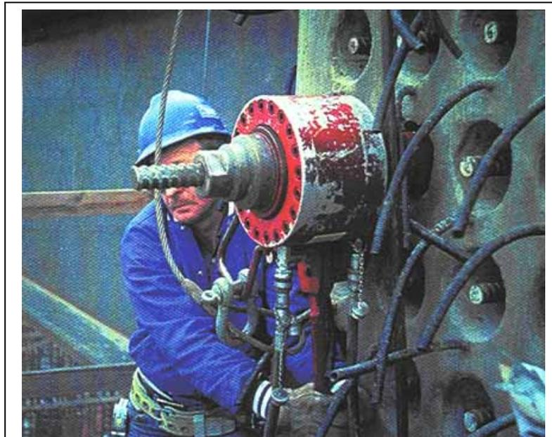
Photo 7-3 – High Strength Bar Stressing Operation.
