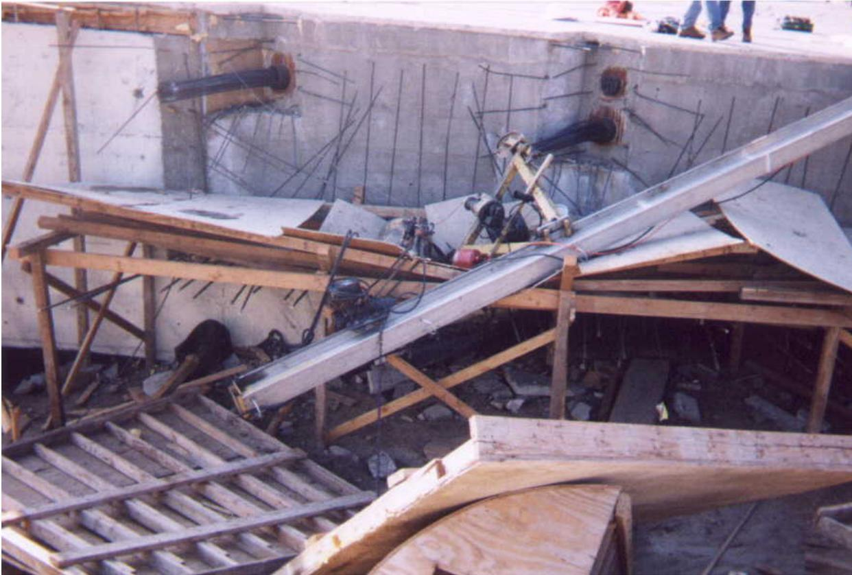
**Photo 1-1 – Example of Failure During Prestress Operations.**
