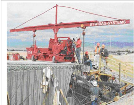
Photo 7-1 – DSI Post-Tensioning Operation.
