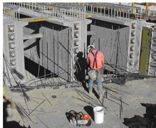
Photo A-2 – AVAR Spliced Girder Stressing.
