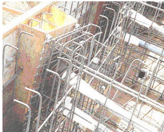
Photo A-4 – DSI Anchorages and Block-out.
