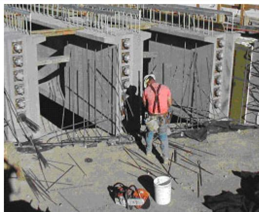
Photo A-2 – AVAR Spliced Girder Stressing.
