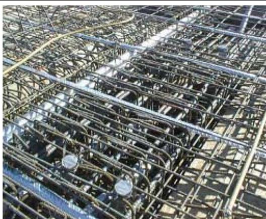
Photo 3-5 – Transverse Ducts in Place.
