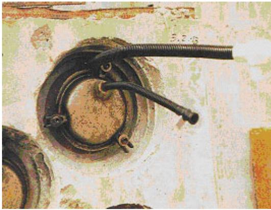
Photo 9-3 – Grout Cap and Tubes in Place. |
