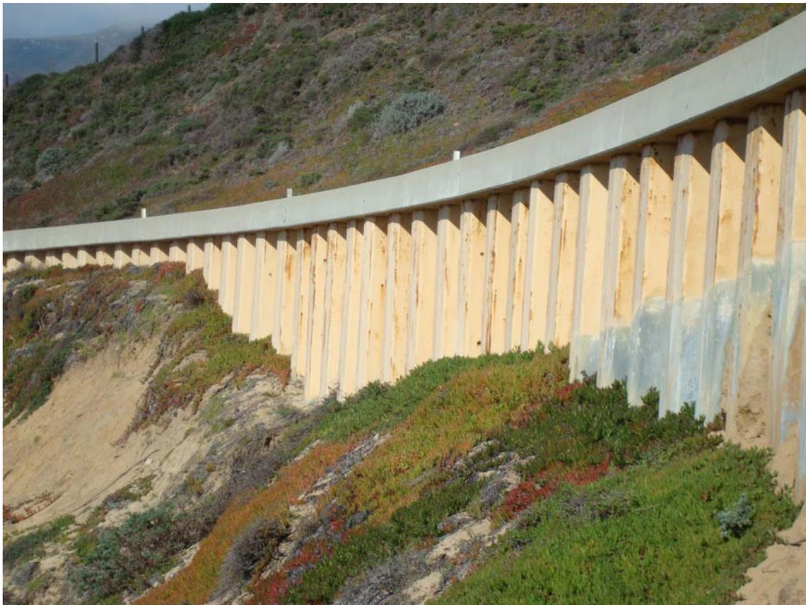
Figure 6-1. Sheet Pile Wall with Cap Beam
