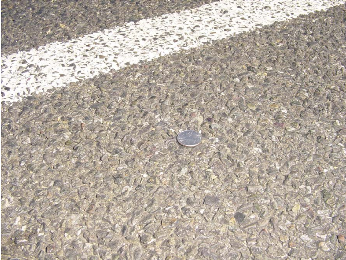
Figure 2-2: Photograph of OGAC Overlay
