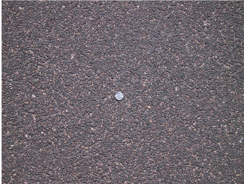
Figure 6-73: Photograph of asphalt rubber friction coarse (ARFC) pavement
