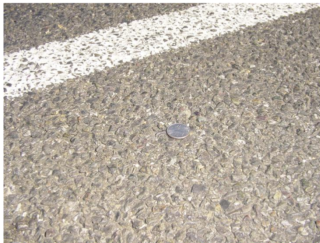
Figure 6-49: Photograph of I-80 Davis OGAC overlay
