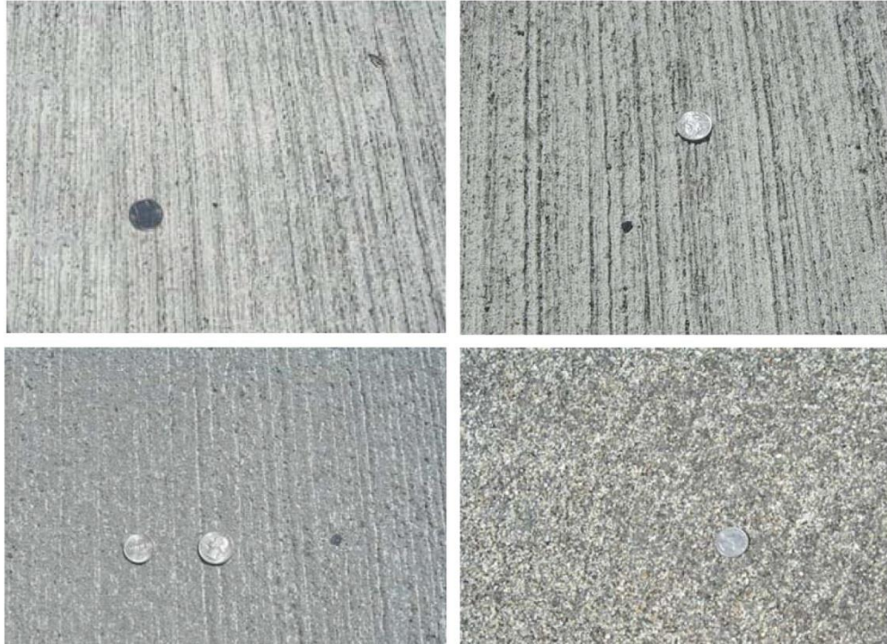
Figure 6-41a: Photographs and Summary of Pavements Measured on Bridge Structures in California
