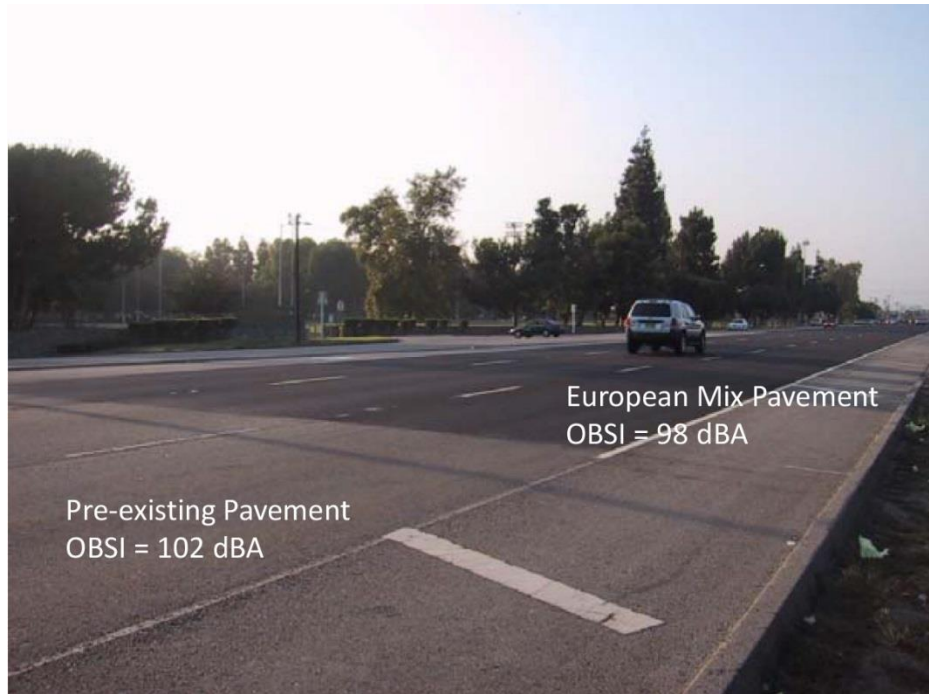
Figure 6-22: Site photo of SR 19, indicating pre- and post-construction surfaces
