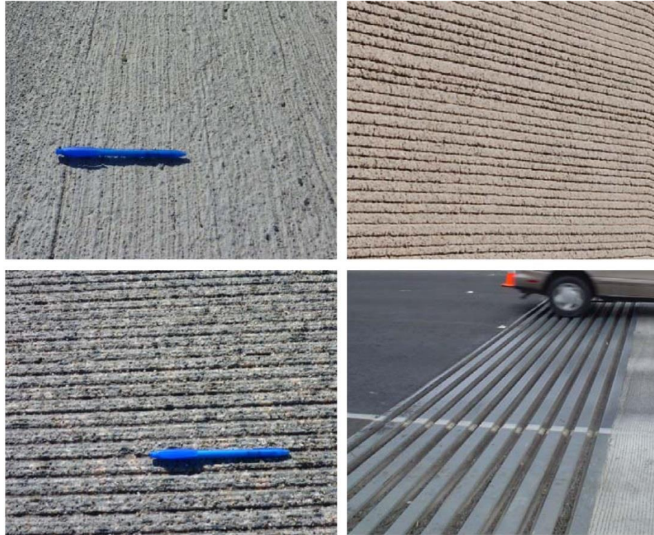
Figure 6-41b: Photographs and summary of pavements measured on bridge structures in California
