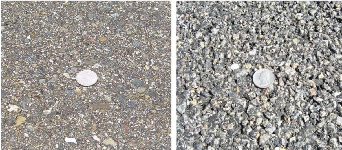
Figure 6-24: Photographs of Shasta 299 pavement surfaces Left: Type A dense grade asphalt concrete (DGAC). OBSI = 103.0 dBA (SRTT) Right: Rubberized asphalt concrete (RAC-O). OBSO = 99.7 (SRTT)
