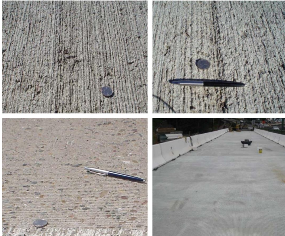
Figure 6-41c: Photographs and summary of pavements measured on bridge structures in California
