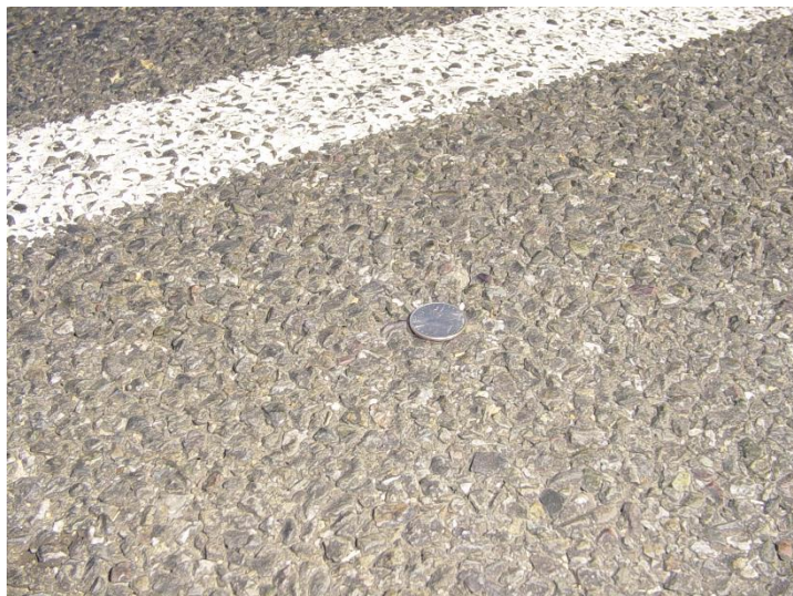
Figure 6-20: Photograph of OGAC overlay on I-80, Davis, California
