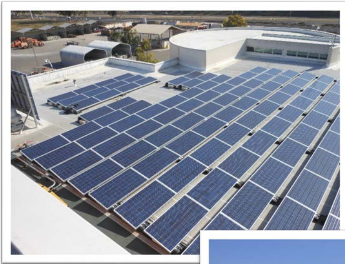
District 12 Transportation Management Center
