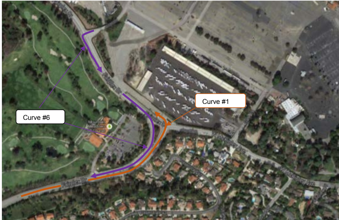
Curves at Entrance and Exit of Racetrack on Fairplex Dr. (Curve #1 & #6)
