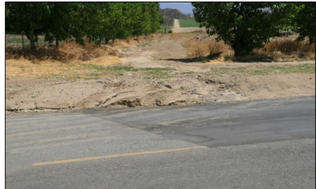
Figure 2.2: Example of road below natural ground level.
