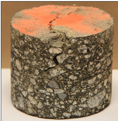
Figure 3.44: Partial-depth top-down crack (caused by low temperatures).
