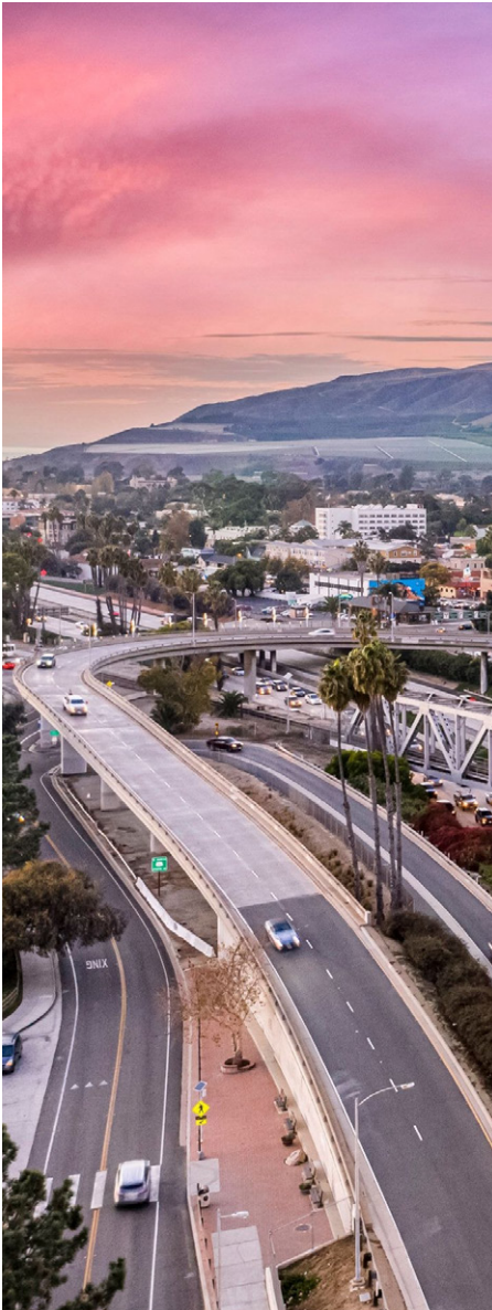
Highways interchange near Ventura at sunset.
