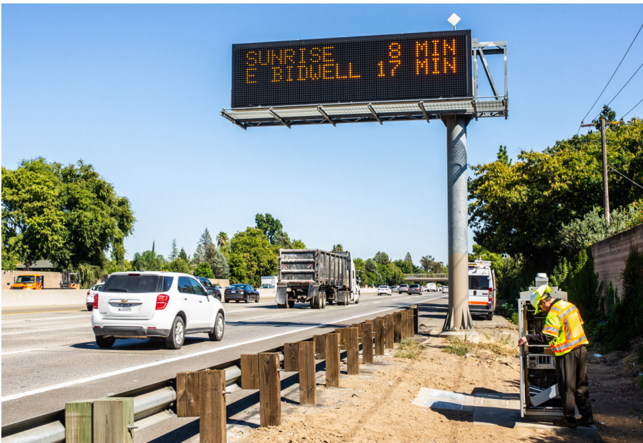
A Caltrans employee inspects a dynamic message sign displaying current travel time messages to motorists.
