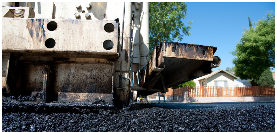
Road paving using rubberized asphalt, a new recycled tires technology.
