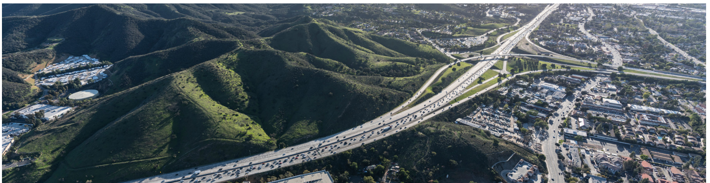
Aerial view of the Ventura Freeway near Thousand Oaks, California.
