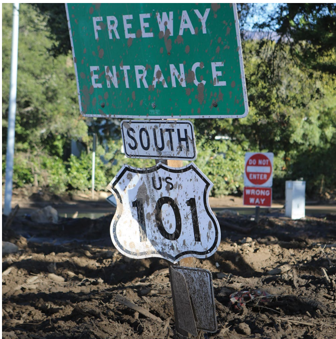
The Montecito mudslide looked like an impenetrable mess at first, but Caltrans and first responders had US 101 open in two weeks.
