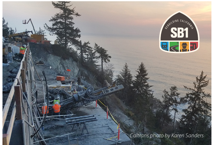
On US 101 in Del Norte County, crews perform repairs on the highway at what's known as Last Chance Grade south of Crescent City.
