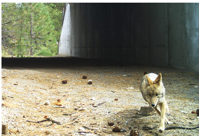
At certain crossings, such as this large culvert, Caltrans has installed trail cameras to see if animals use the passages. This coyote did.
