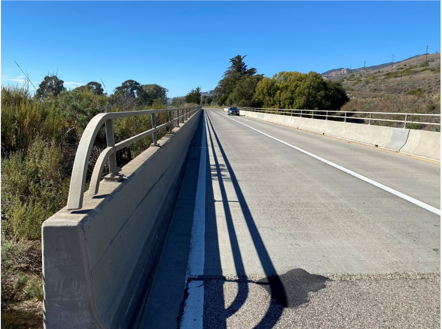
Looking northbound at the Arroyo Quemada Bridge
