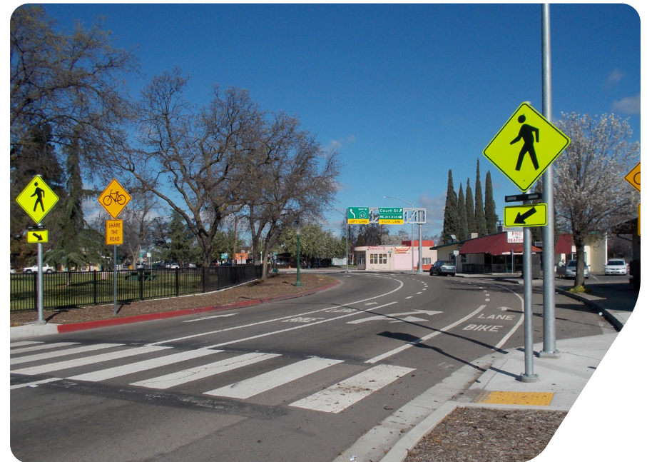
SR 63 at Lincoln Oval Park in Visalia features bicycle lanes and a pedestrian-activated crossing beacon.
