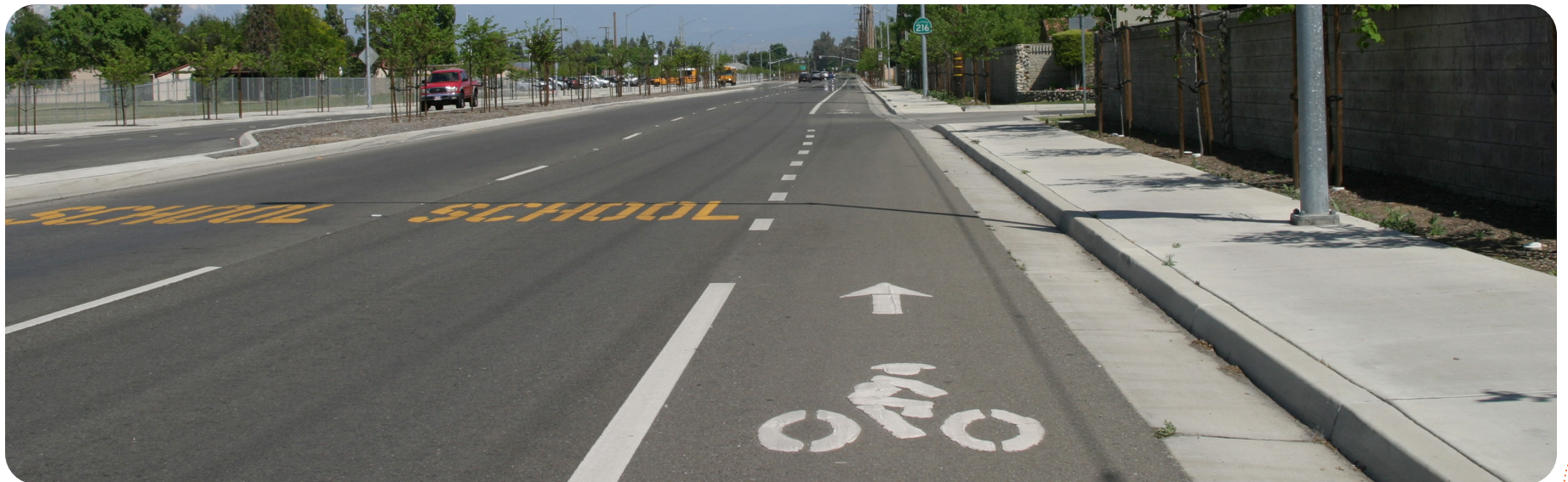
A wide sidewalk, driver-oriented signage, and a wide bicycle lane along SR 216 in Visalia help improve safety for children walking and bicycling to nearby schools.
