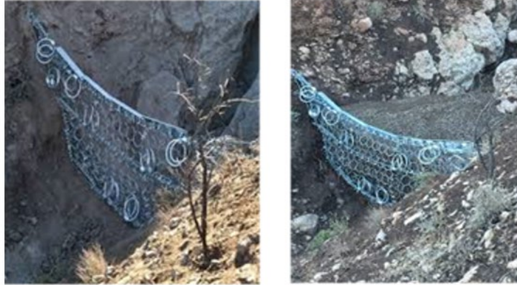
FIGURE A- 4: EXAMPLE OF DEBRIS FLOW DETENTION FENCING AS DESIGNED (LEFT) AND HOLDING BACK DEBRIS FLOW (RIGHT)
