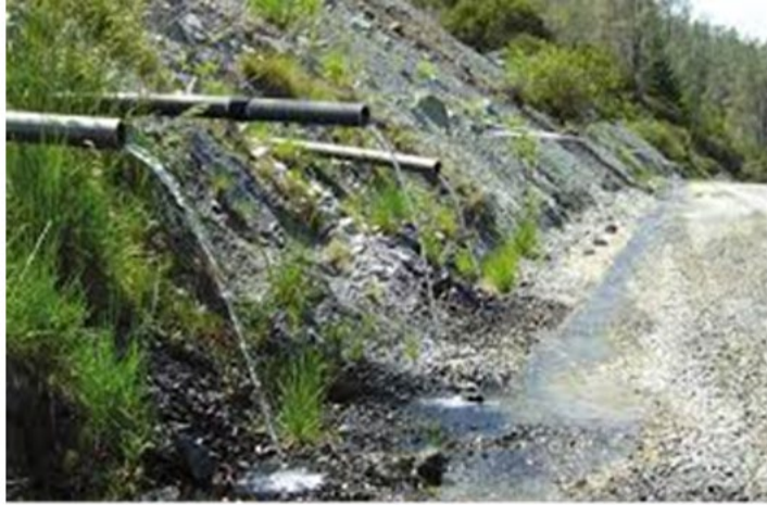
FIGURE A-5: DRAINAGE TO STABILIZE SLOPE
