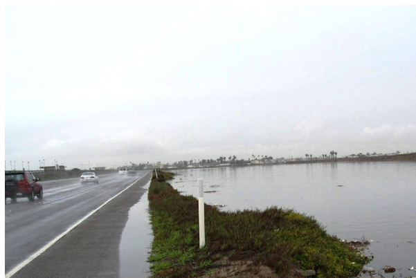
WATER ENCROACHMENT ON SR 1, DISTRICT 5
