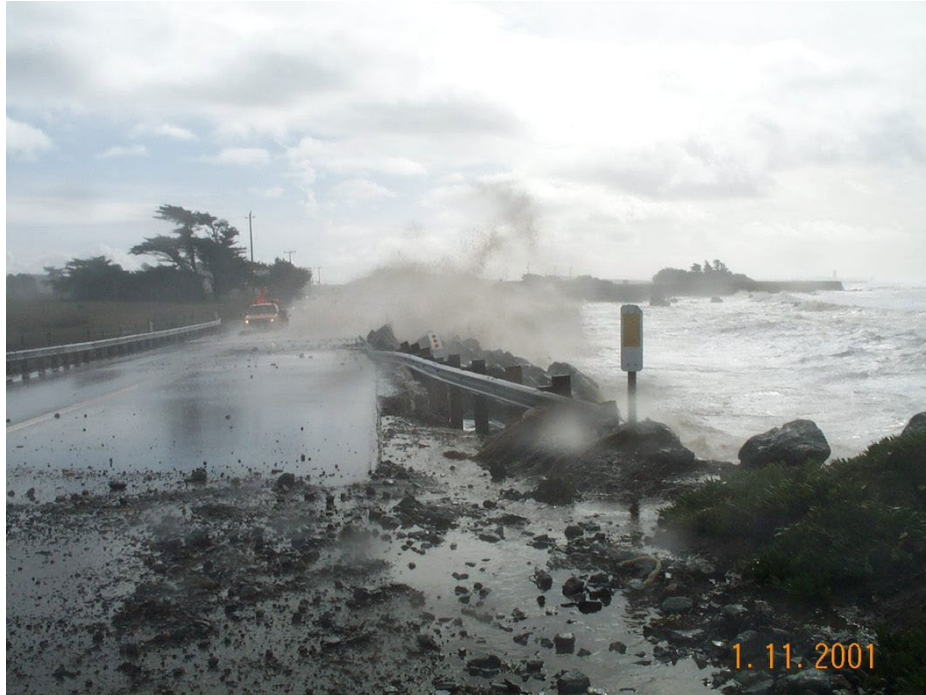
SR 1 Prior to Realignment
