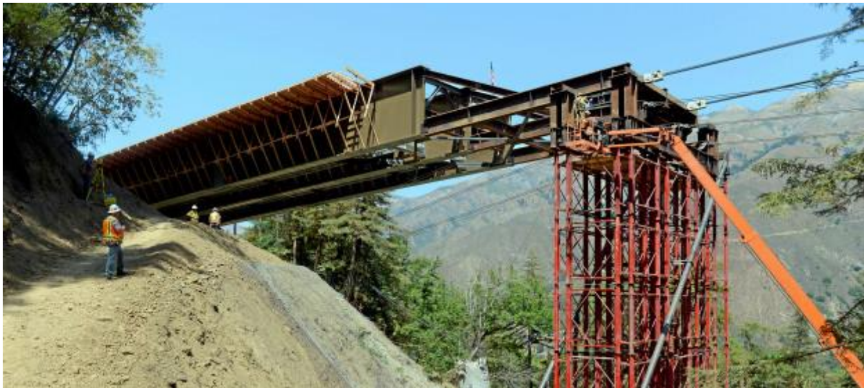
Pfeiffer Canyon Bridge Launch
