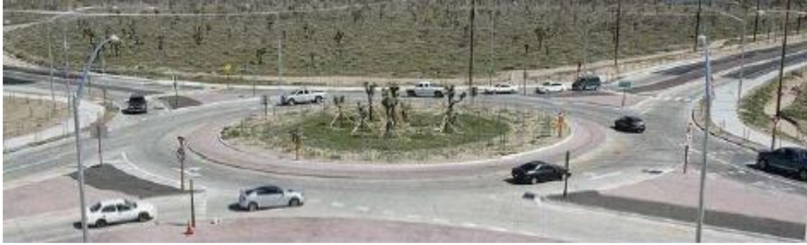
Roundabout on Route 138 in Palmdale
