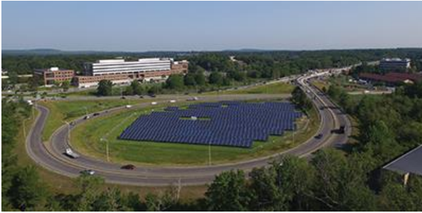
MassDOT-installed solar panels in the ROW at Exit 13 North on I-90 in Framingham, MA
